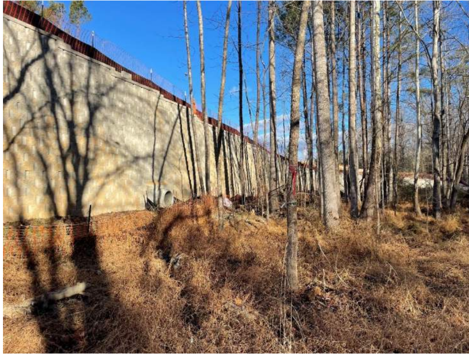
Photo C.2: New stormwater pipes from South Creek
