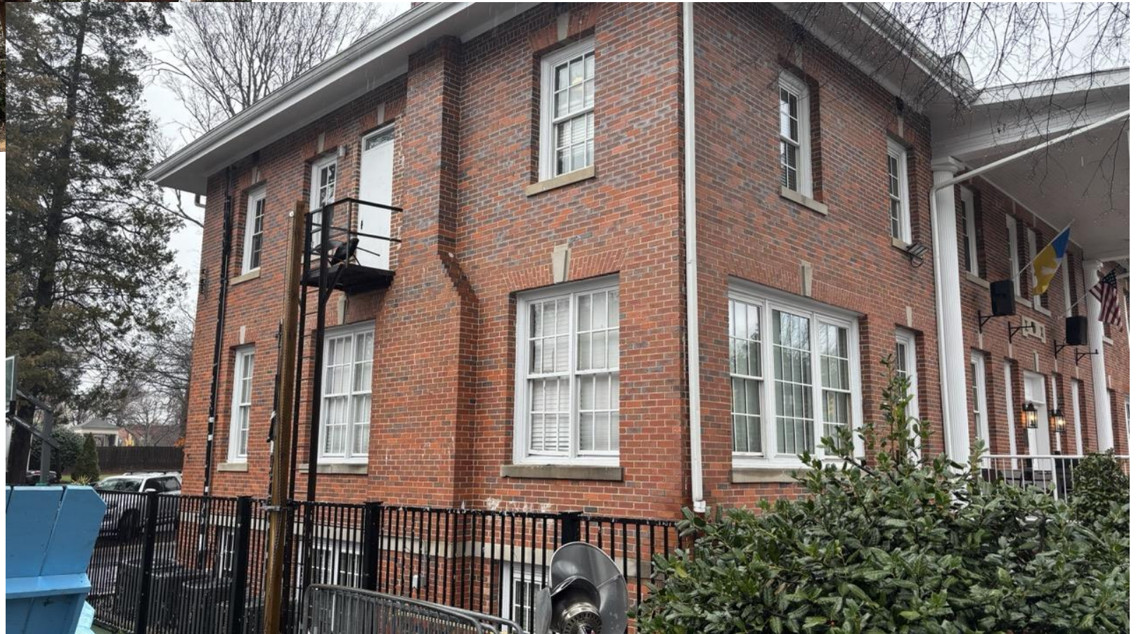
West side – existing ladder fire escape
