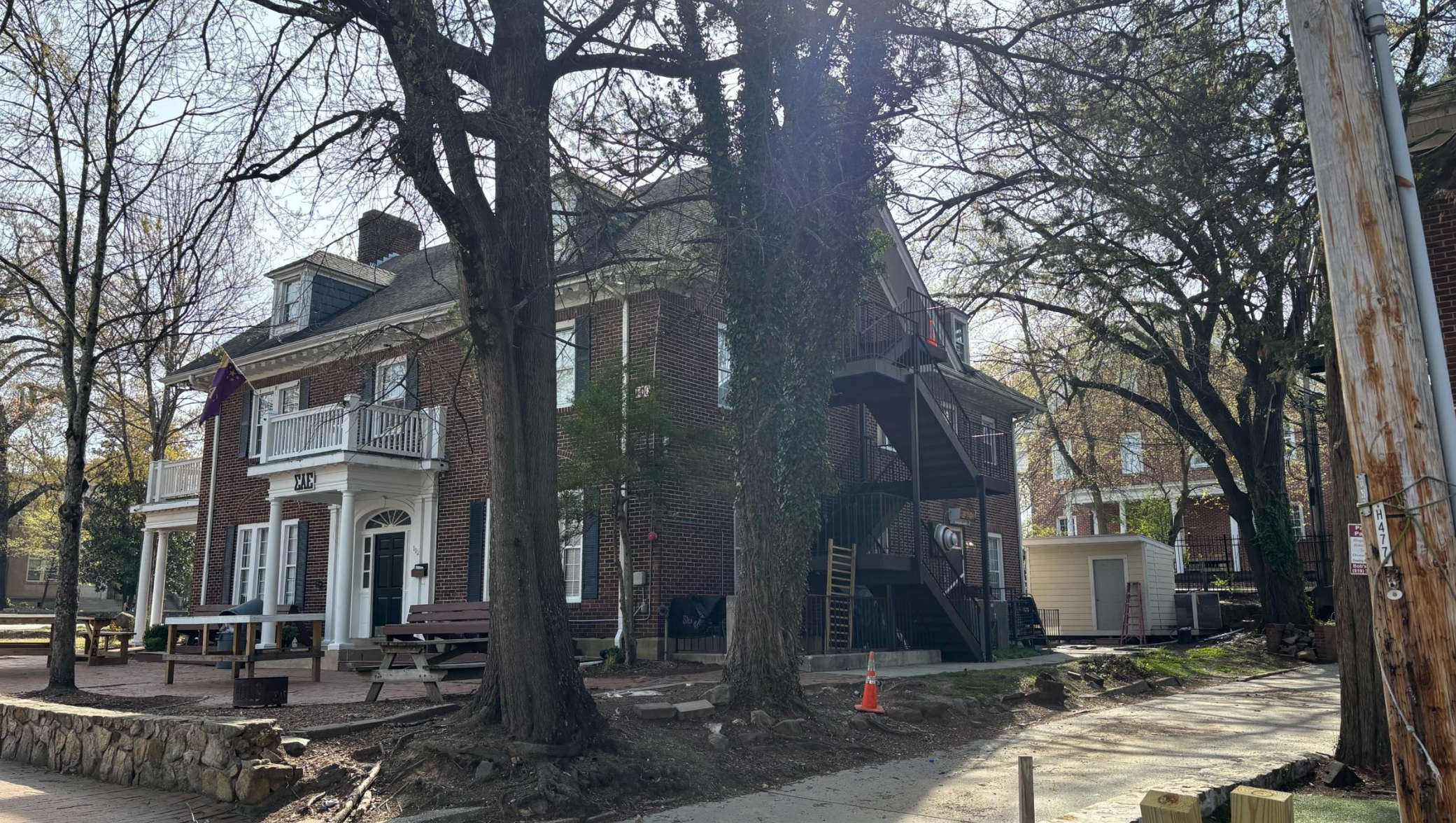
Another house on fraternity court with a full fire escape staircase
