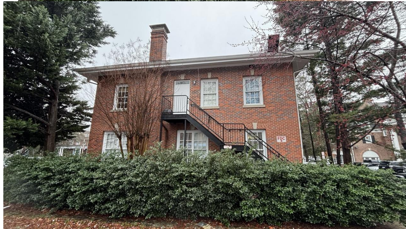
East side – existing fire escape stairwell
