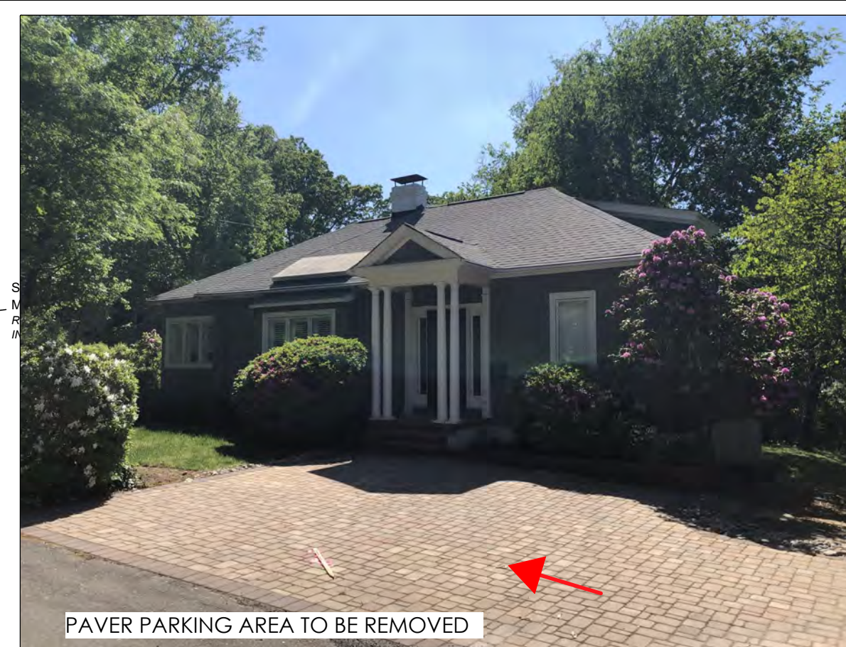
PAVER PARKING AREA TO BE REMOVED
