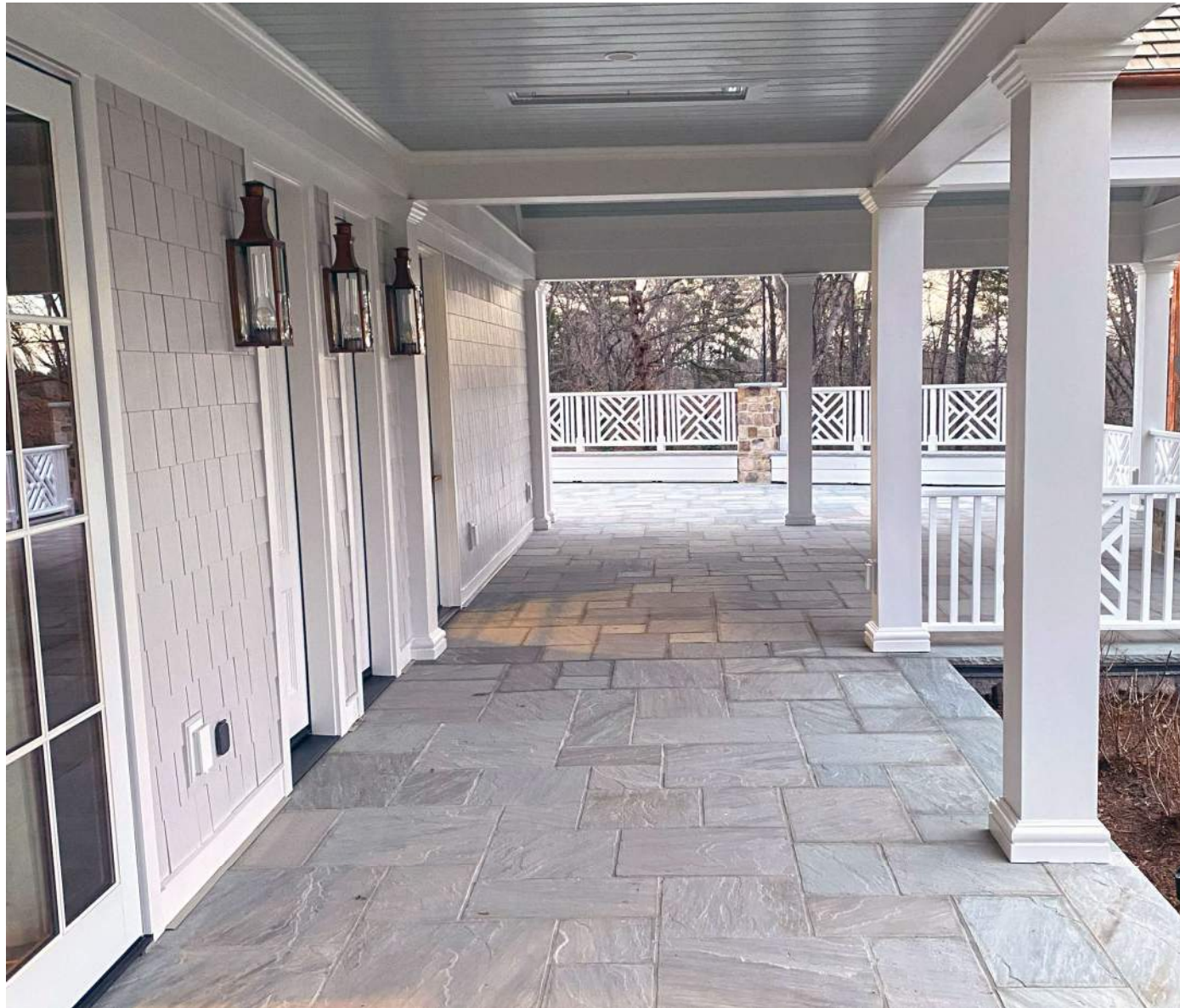
-Example of bluestone porch material, hardie-shingle siding, HB&G columns, and Bevolo light fixtures to be used
