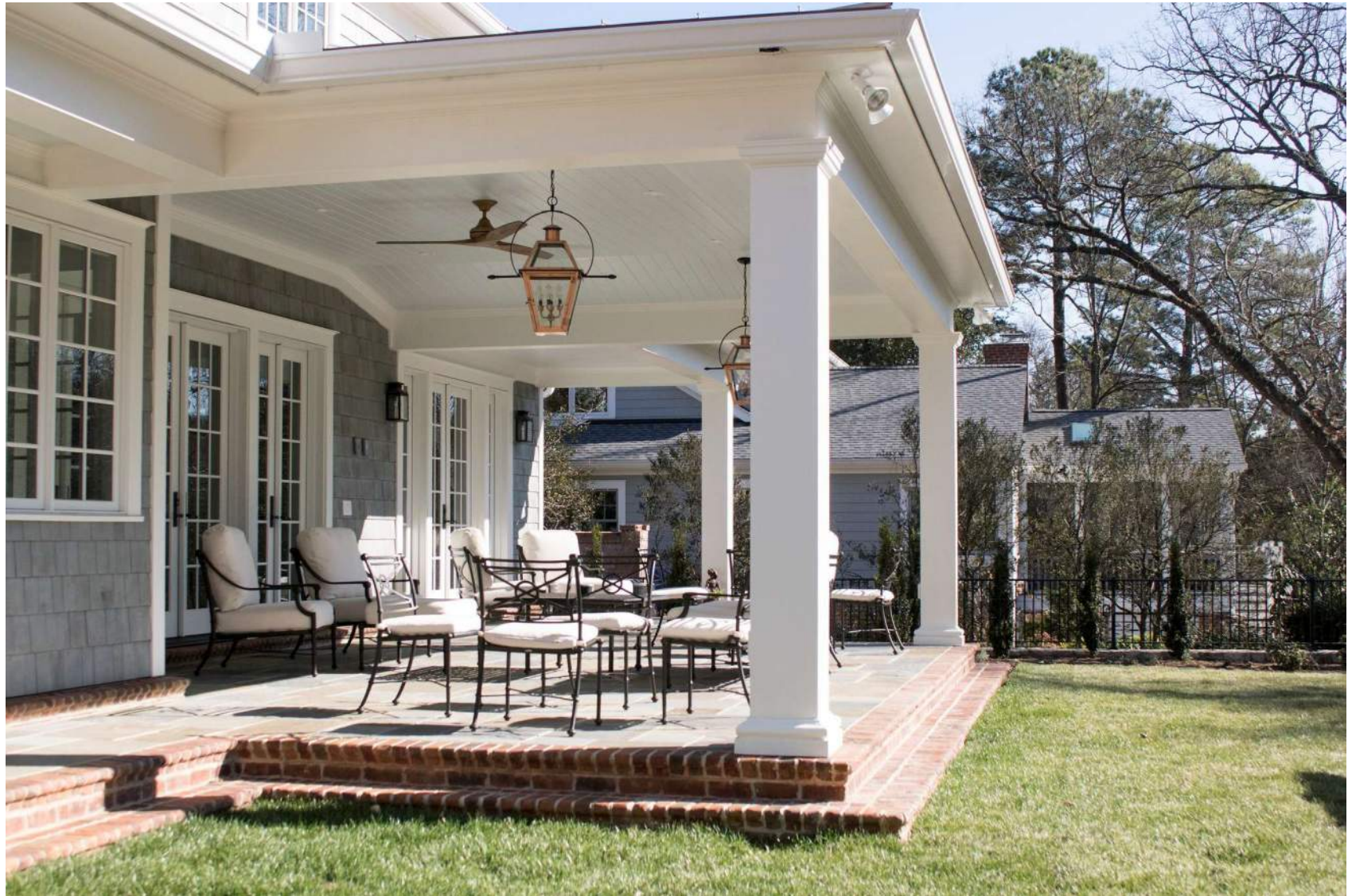
Porch precedent at 704 Gimghoul showing bluestone paving, HB&G composite columns, K-style gutters, a Bevolo French Quarter hanging lantern, and Bevolo Williamsburg sconces flanking the entry.
