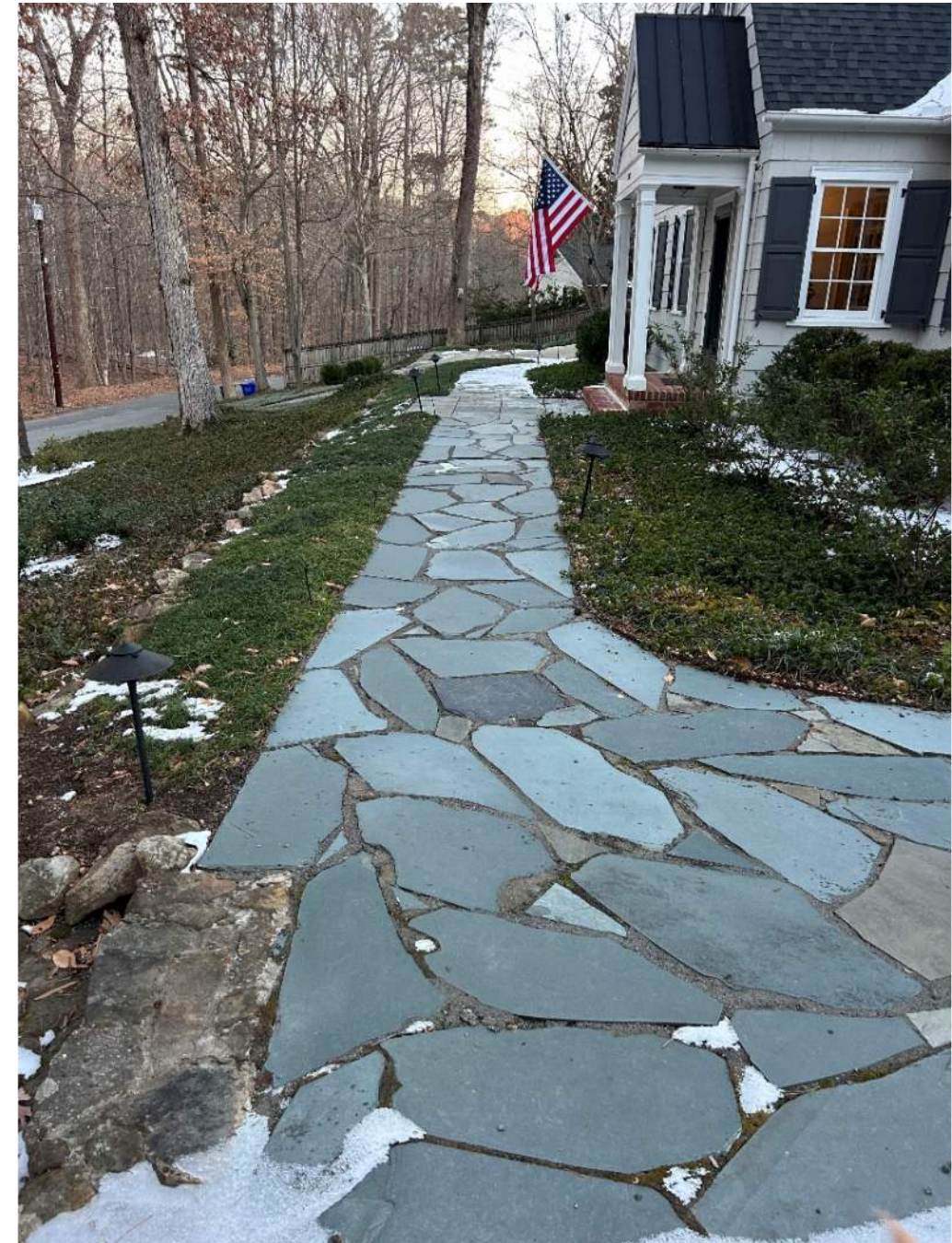
Existing Slate Walkway looking North (to be replaced with brick)
