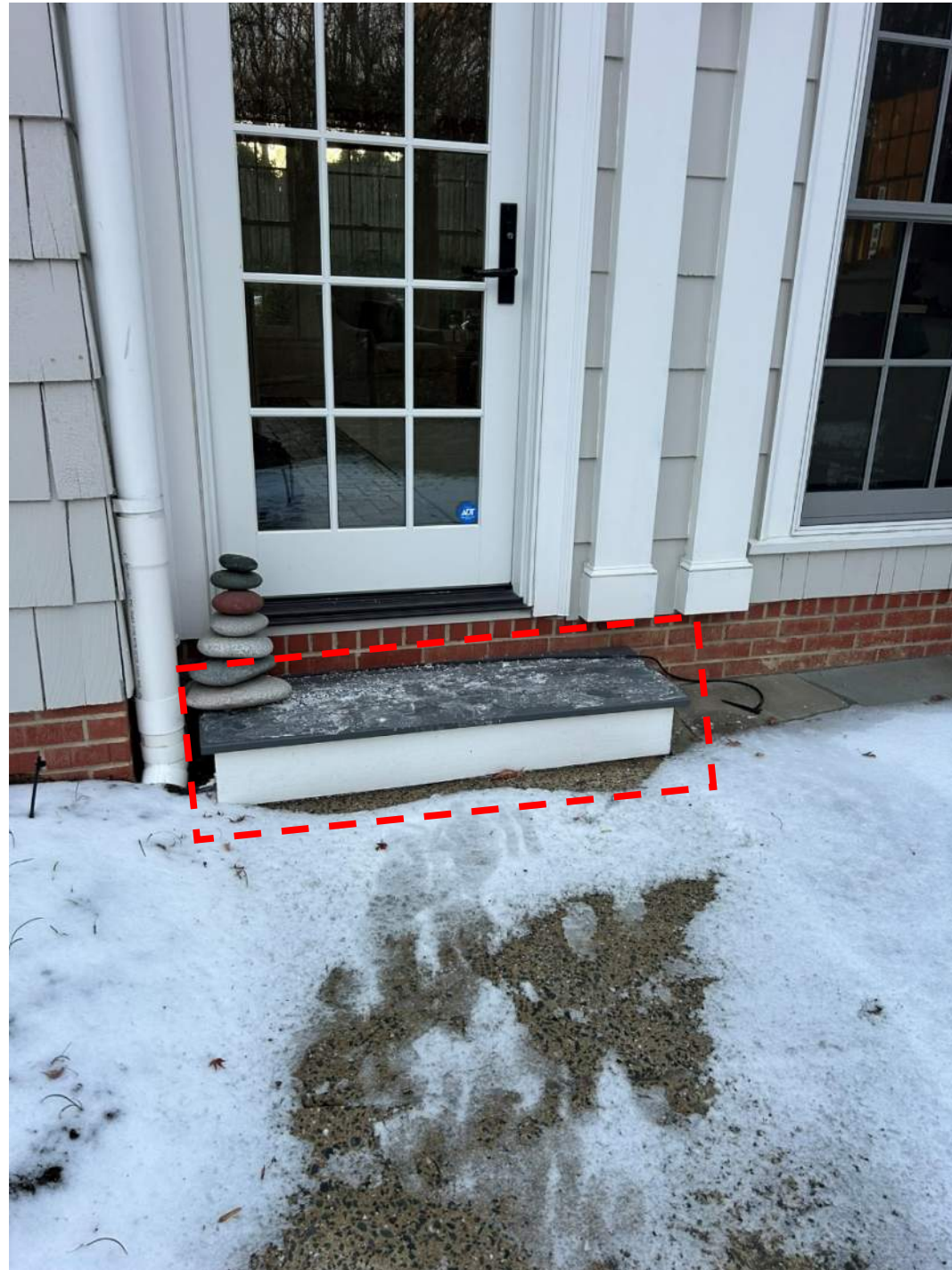
Existing Secondary Step (to be replaced with brick stoop)
