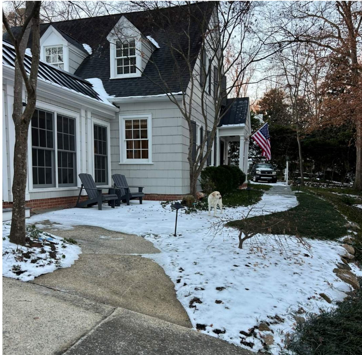
Existing Concrete Walkway looking South (to be replaced with brick)
