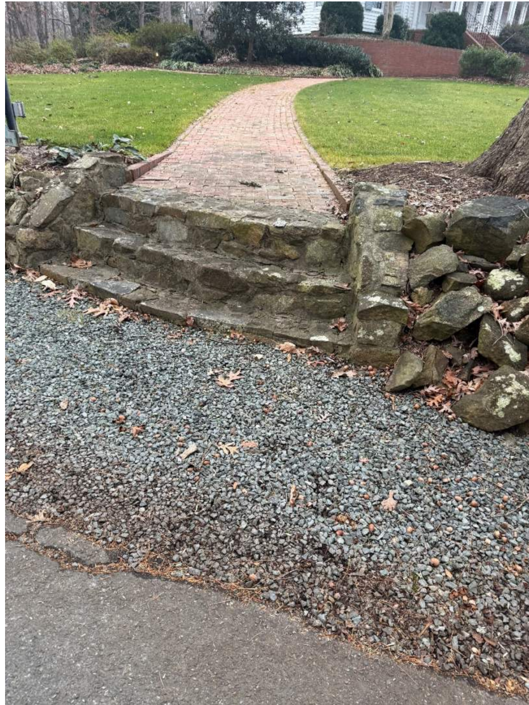
246 Glandon Drive Stone Steps and brick walk in loose stone wall
