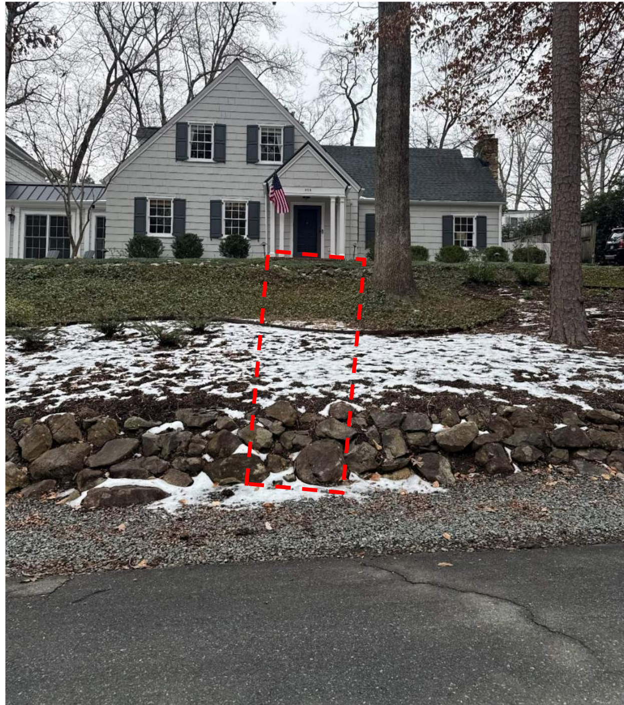
View from Glandon Drive looking at location of new walk and stone Steps
