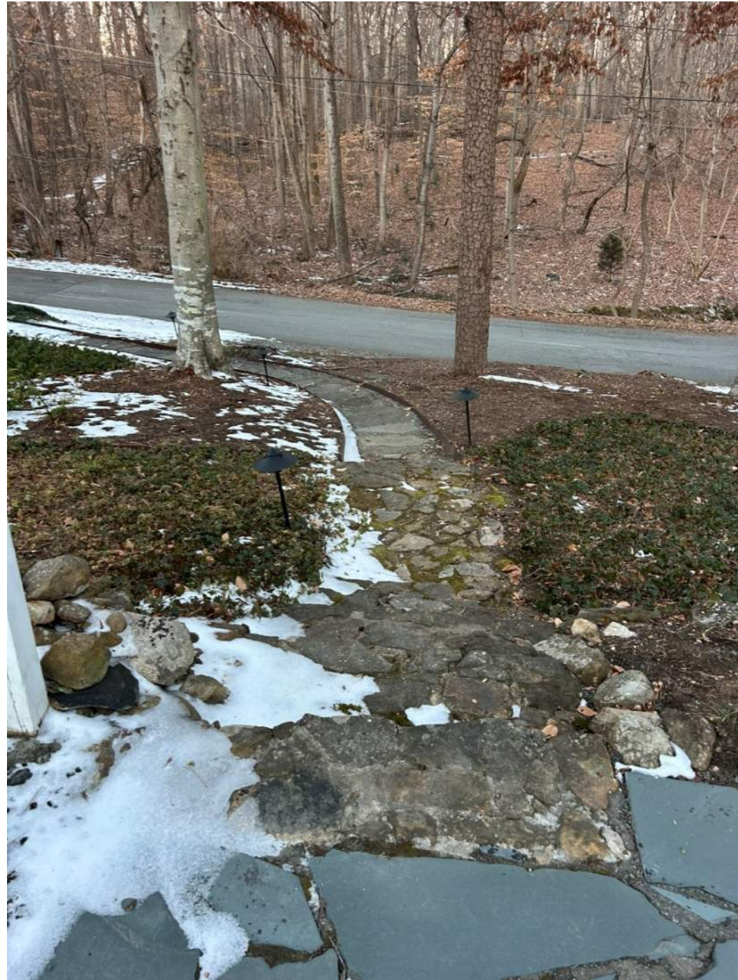
Existing Stone steps and walk looking West (to be removed)
