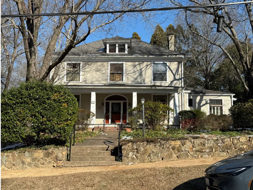
PHOTO 25: Context—house across the street to the northeast @ 214 N. Boundary St.
