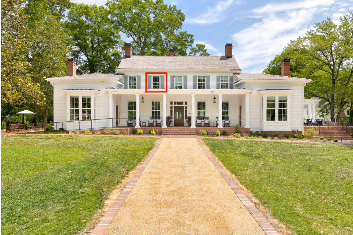
PHOTO 11: Proposed replacement windows of the same kind were approved by the HDC for installation on the North Carolina Study Center.
