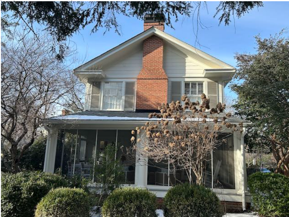
PHOTO 2: South elevation. Both 6-over-6 double-hung windows seen here are proposed to be replaced. The French door on the porch (see Photo 9) is proposed to be replaced as well.
