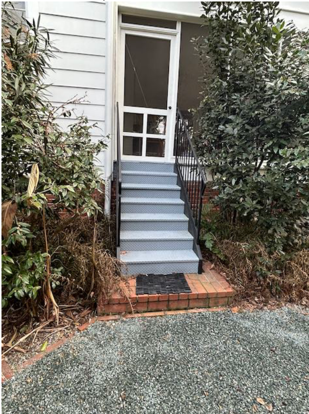
PHOTO 14: Wood stair to rear yard from southern screened porch.
