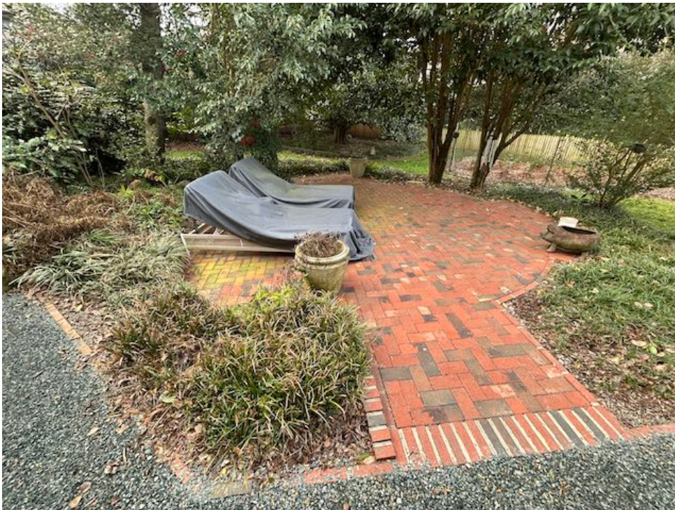
PHOTO 16: Brick patio (seen in Photo 15) detail.
