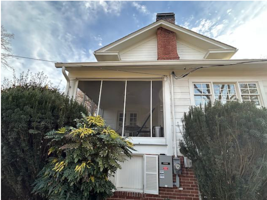
PHOTO 6: North elevation. Two six-over-six double-hung windows on the upper floor cannot be seen here, but are proposed to be replaced. The French door on the porch (see Photo 10) is proposed to be replaced as well.
