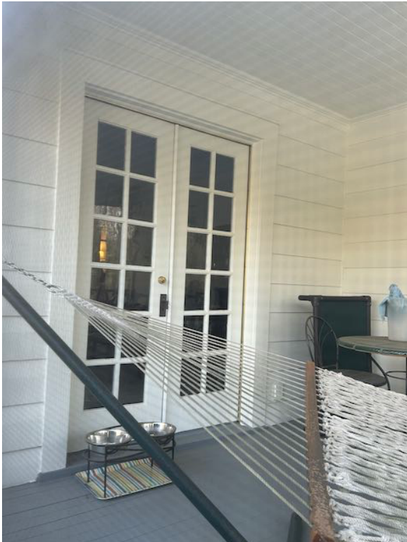
PHOTO 10: Detail of French door onto northern screened porch that is proposed to be replaced.
