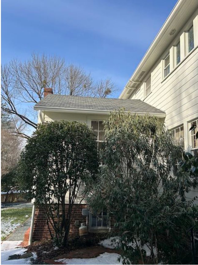
PHOTO 3: South elevation of rear bump-out. A cross-gabled addition is proposed on the west side of this bump-out.
