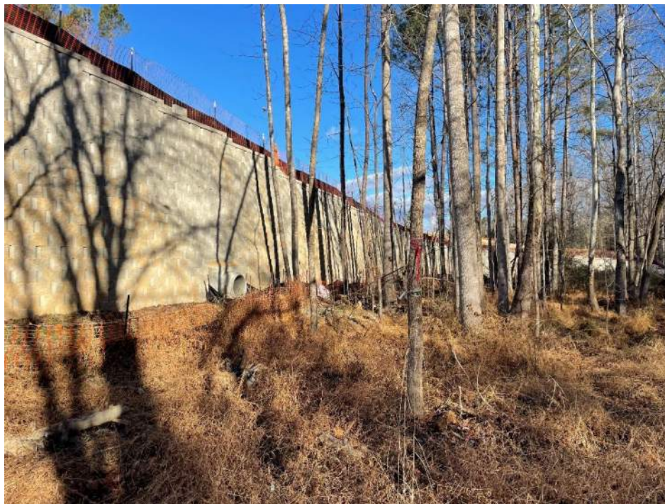
Photo C.2: New stormwater pipes from South Creek
