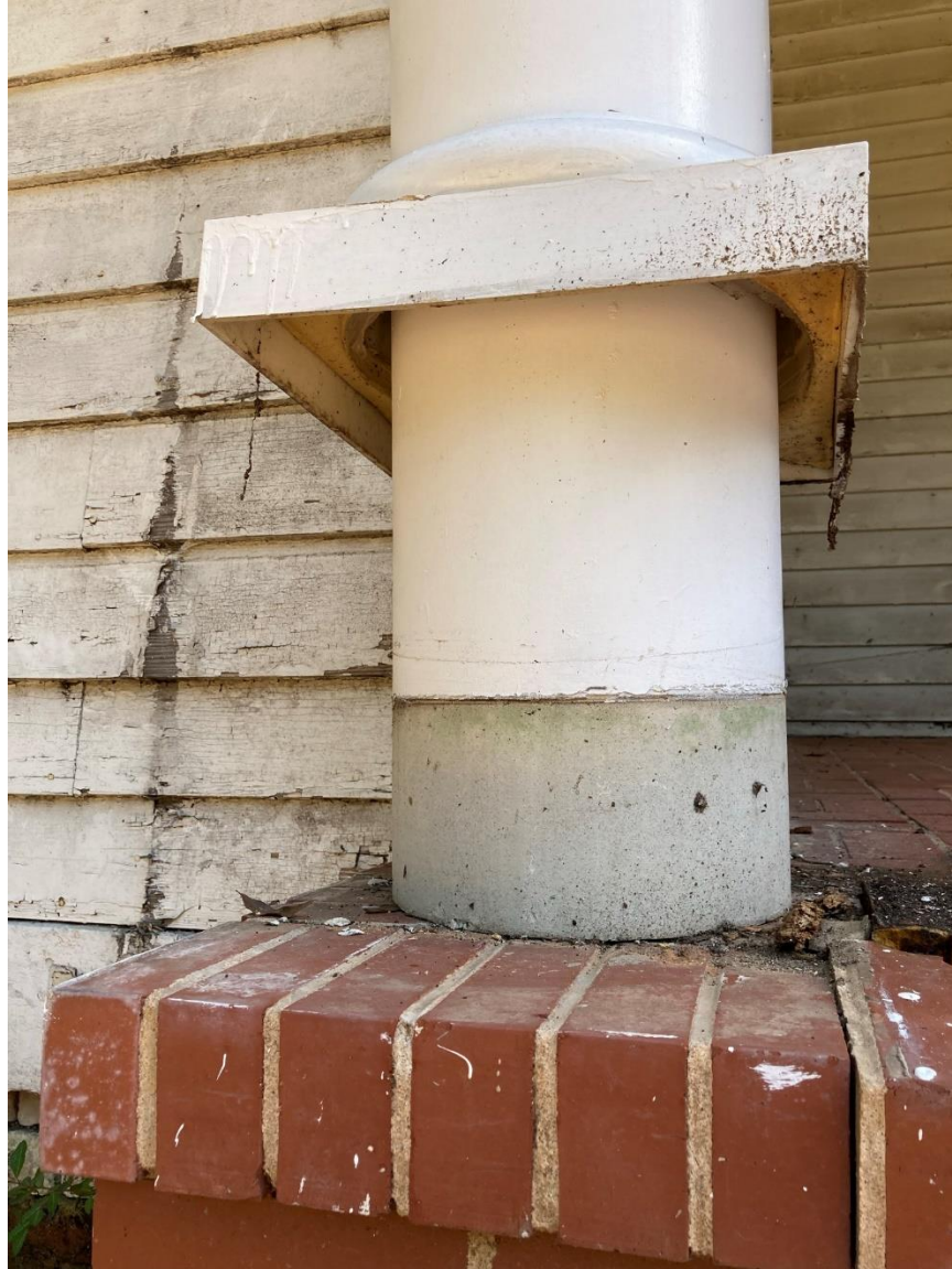
Column N3 base. Furniture-grade structural foam base, lifted up to show how it slides onto shaft.
