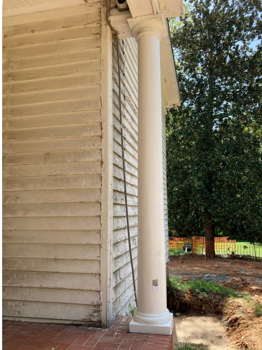
Column S3. Perhaps an original from the 1920's renovation, however wood shaft is narrower than other wood shafts, capital is wood; the base is a replacement furniture-grade structural foam base.
