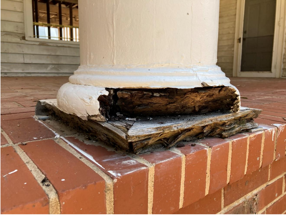
Column S1 base. Shows significant water damage. Metal standoffs, at the four corners of the base, were employed at some point in the past in an attempt to allow air and water circulation under the base.
