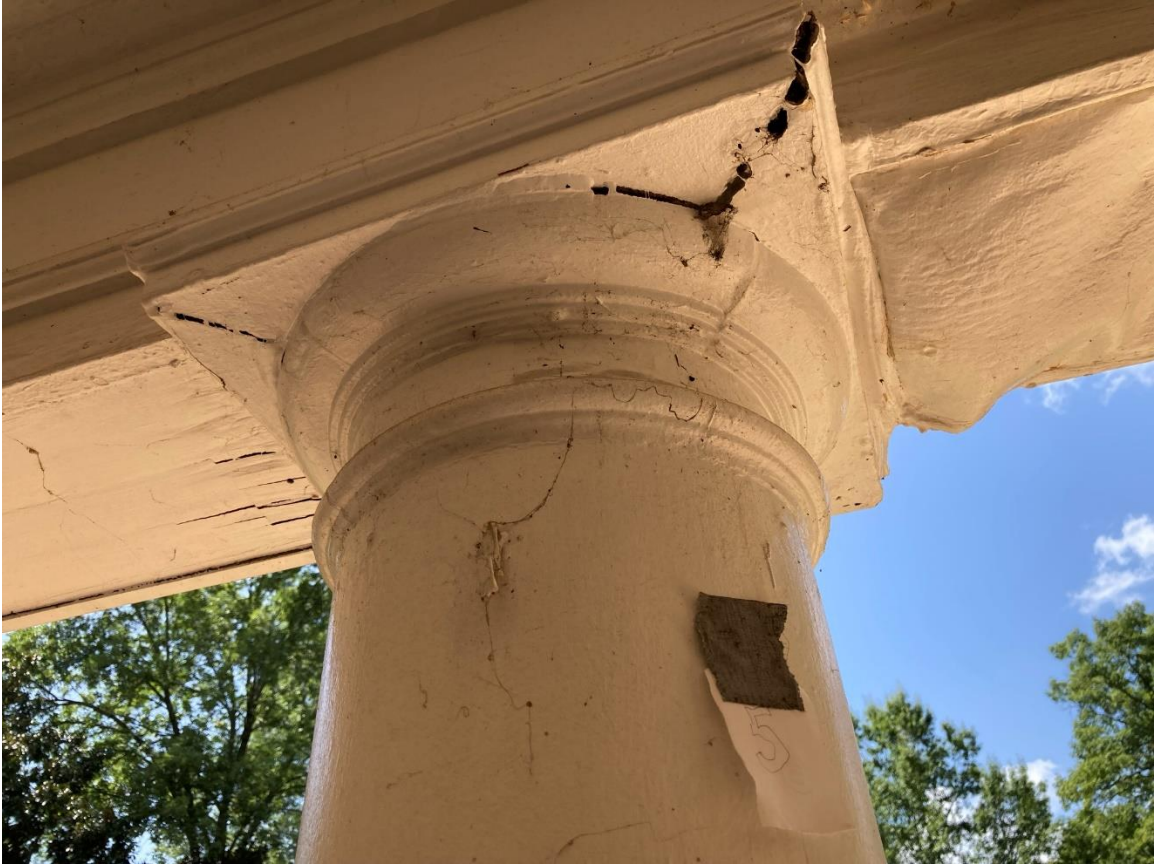
Column S2 capital showing water damage.
