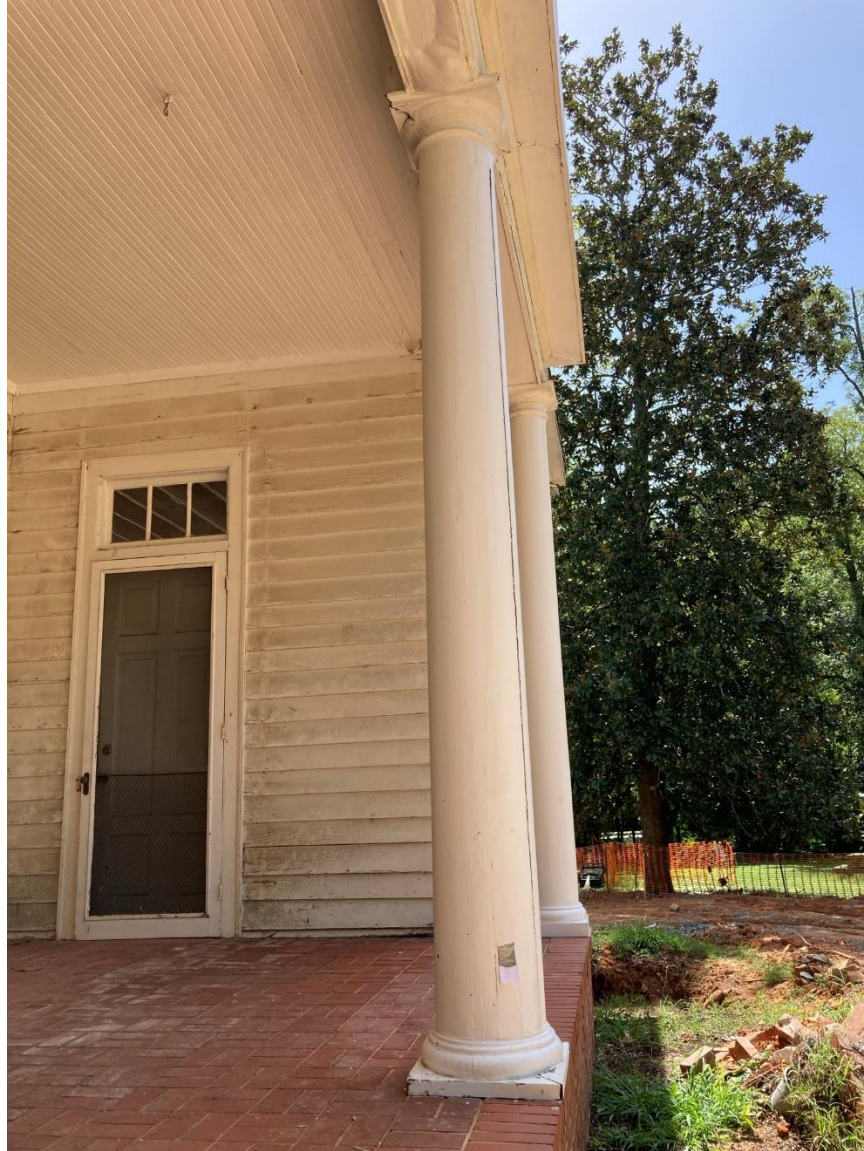
Column S2. Likely an original from the 1920's renovation. All wood. A large split in the finger-jointed wood of the shaft can be seen on the right edge of the column.
