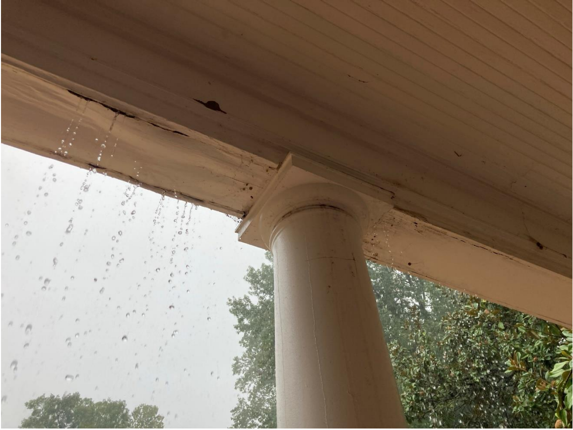
Column N2 capital. Furniture-grade structural foam capital and base do not show any indication of needing repair.
