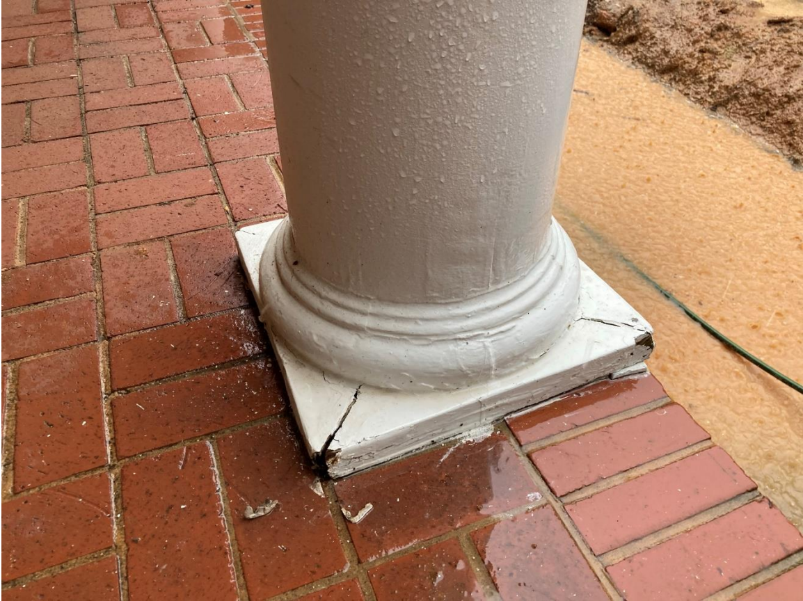
Column N1 base. A screwdriver was able to be pushed well into the wood at the bottom left corner of the base.
