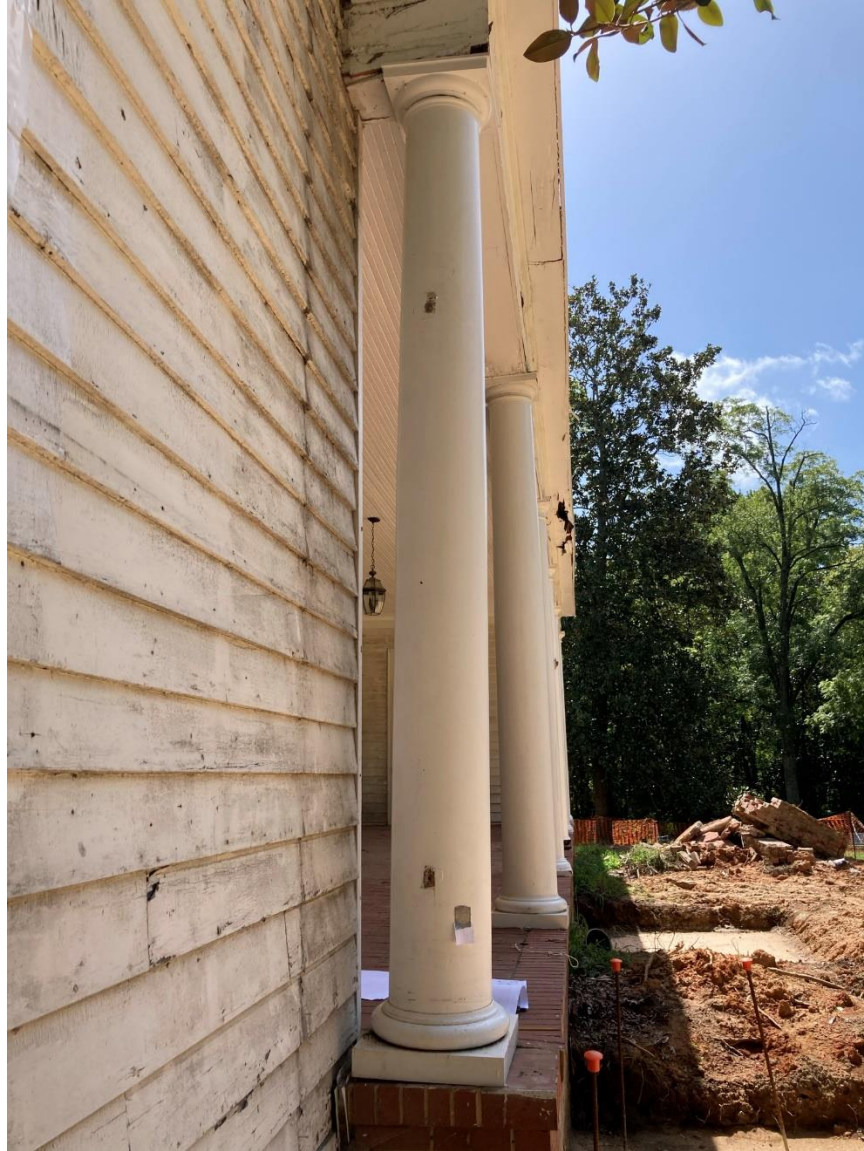
Column N3. Non-original replacement column. Shaft is fiberglass/concrete composite and base and capital are furniture-grade structural foam.
