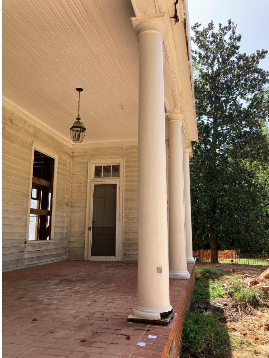
Column S1. Likely an original column from the 1920's renovation. All wood.
