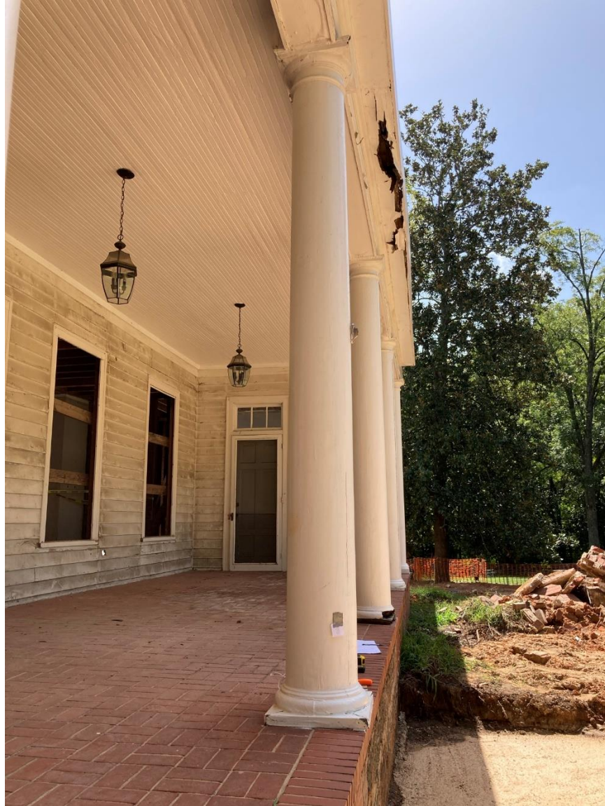
Column N1. Likely an original column from the 1920's renovation. All wood.
