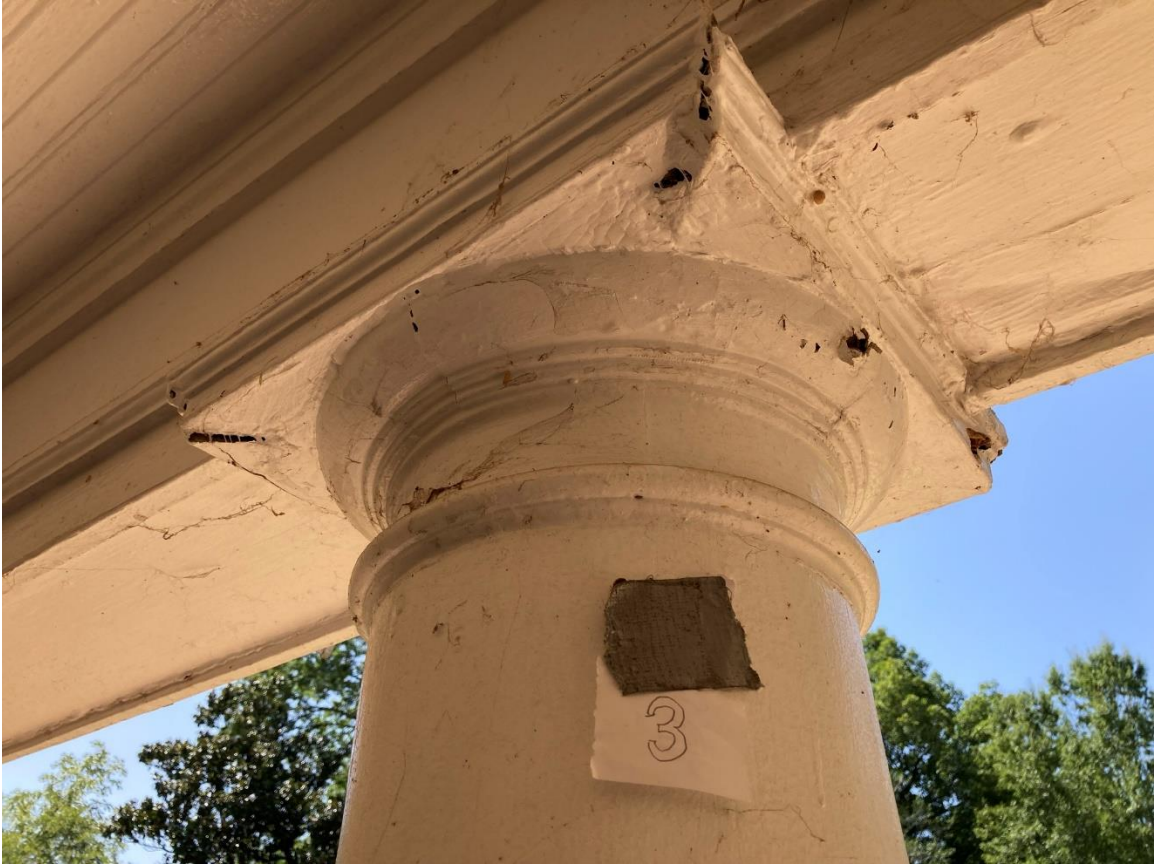
Column N1 capital. Holes in capital indicate where screw-driver probe test was performed and where significant rot was discovered.
