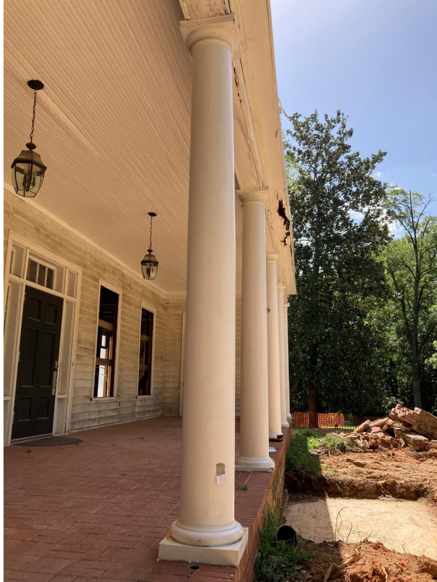
Column N2. Non-original replacement column. Shaft is fiberglass/concrete composite and base and capital are furniture-grade structural foam.
