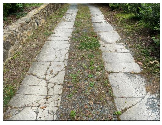
Middle portion of driveway showing deteriorated concrete strips
