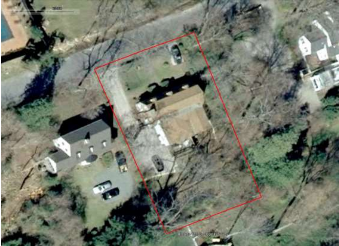
Figure 63 - Satellite Image from 2008 Showing Possible Different Color and Material for driveway and parking pad.
