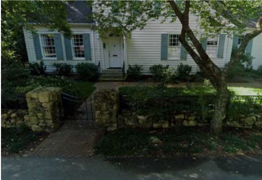
Figure 69 – 520 Hooper Lane – Walkway Finish
