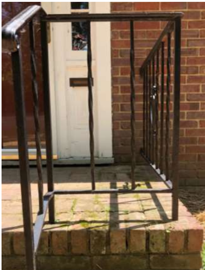
Figure 74 - Existing Metal Railing – Front View
