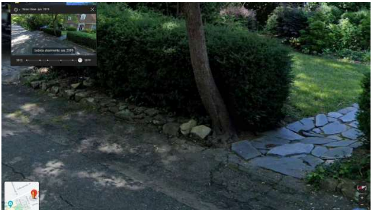
Figure 34 – Street view image from 2019 – Evidence of conditions for fieldstone wall and stone walkway
