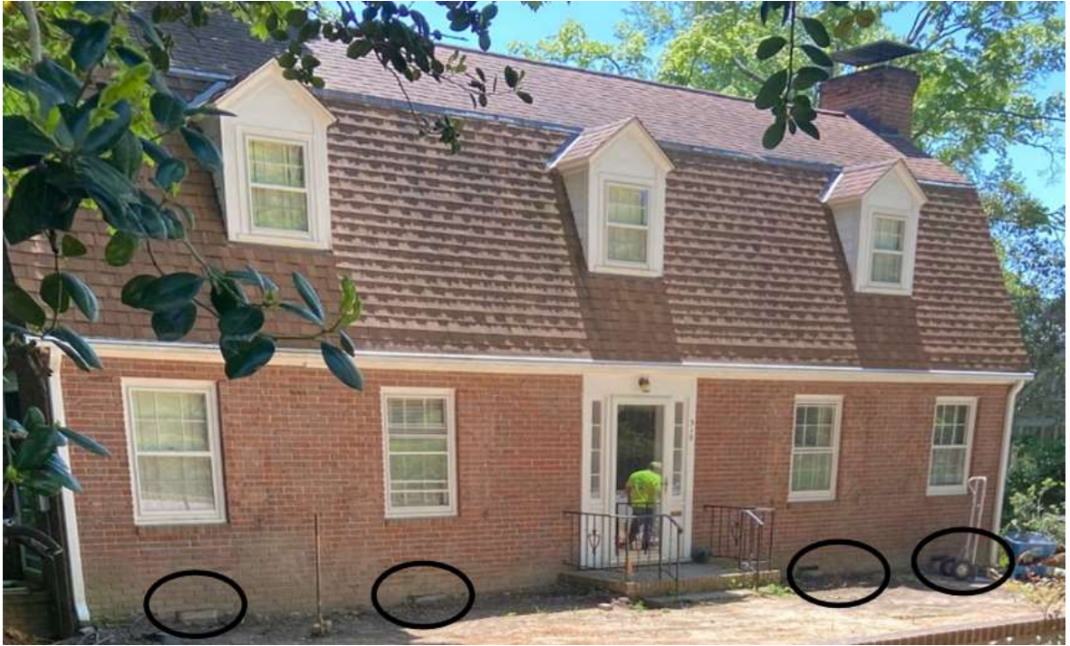
Figure 41 – Basement Vents (Black Circle)
