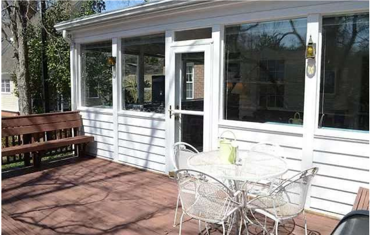
Figure 59 - Rear Deck - White Finishes
