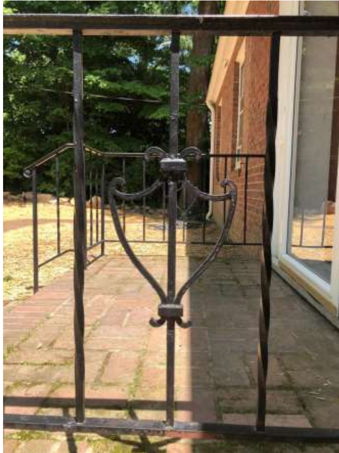
Figure 75 - Existing Metal Railing Side View
