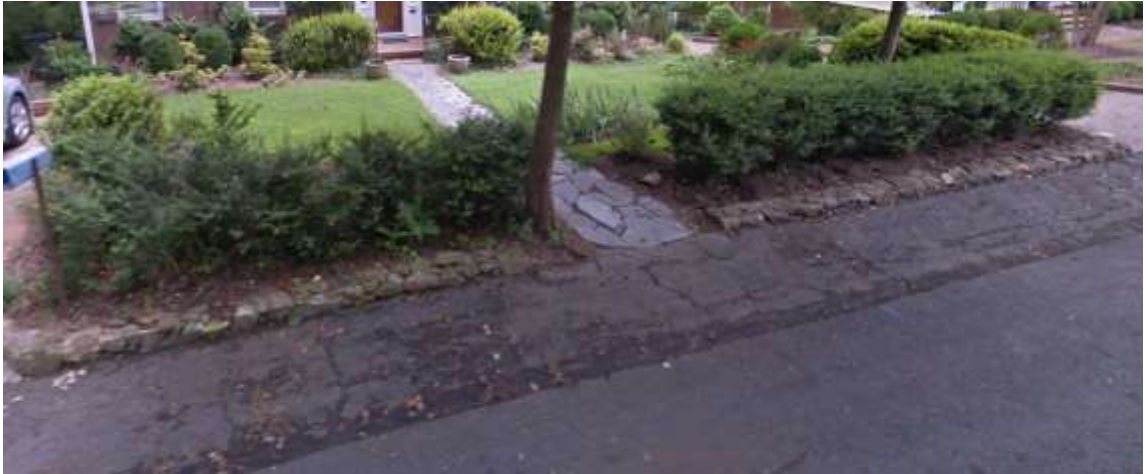
Figure 71 - Existing Fieldstone wall to be replaced.
