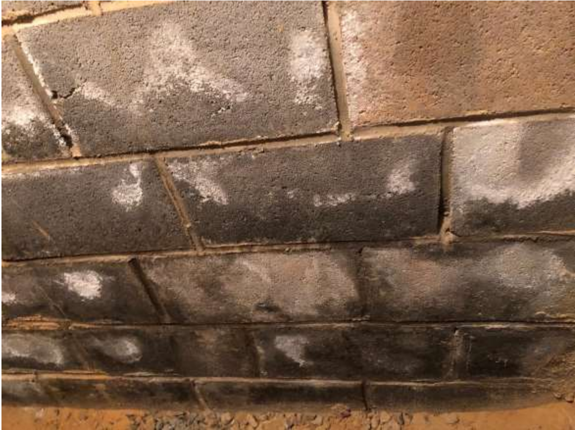
Figure 46 - Appearance of recent block wall installed to contain soil inside the basement.
