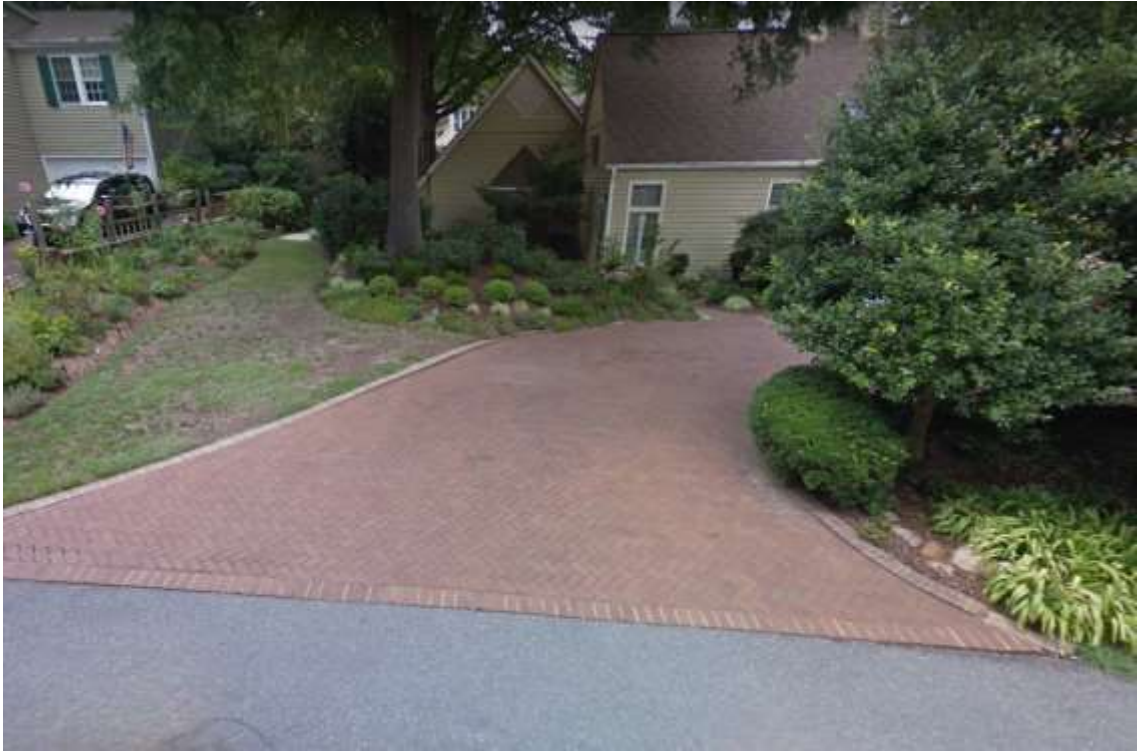
Figure 67 - 521 Hopper Lane - Driveway Finish
