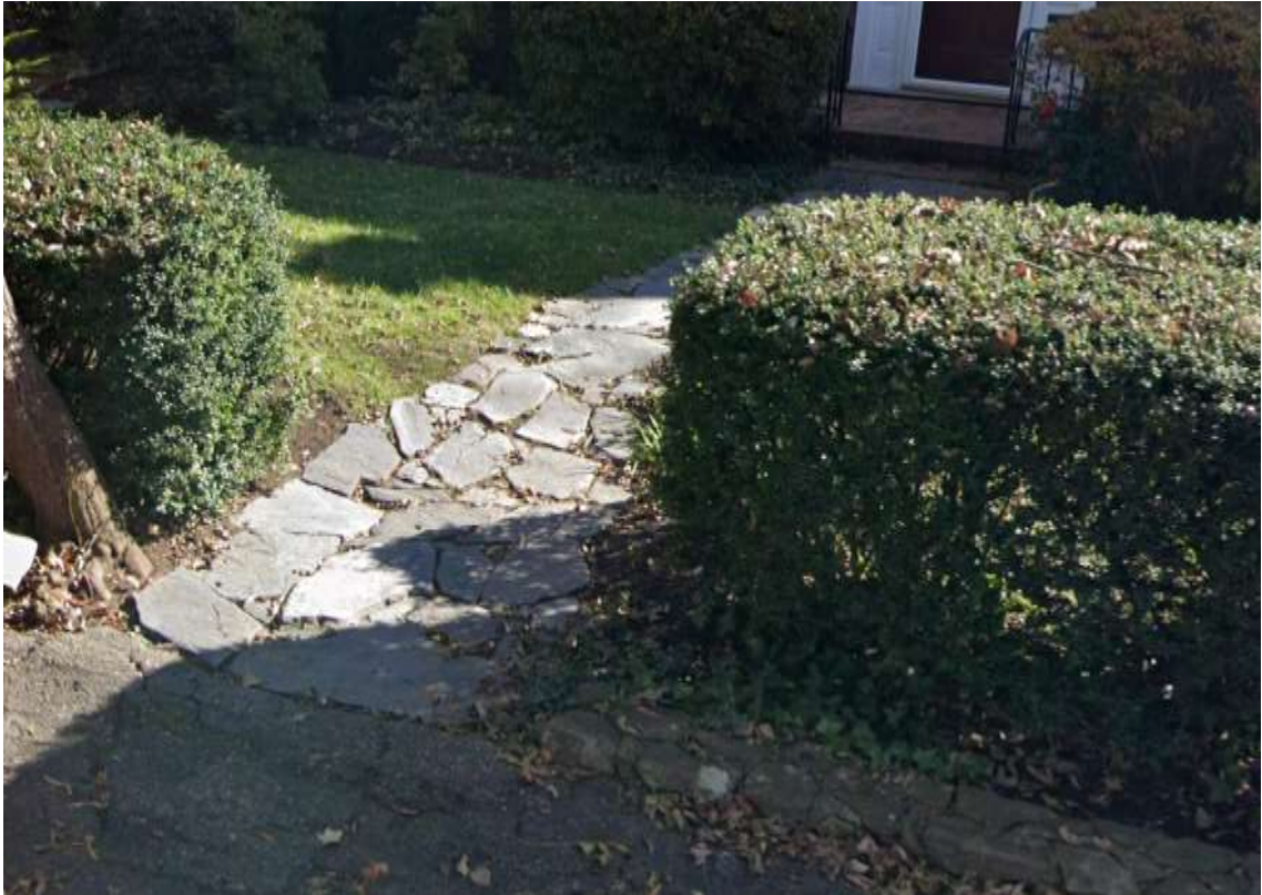
Figure 70 - Previously Installed Stone Walkway
