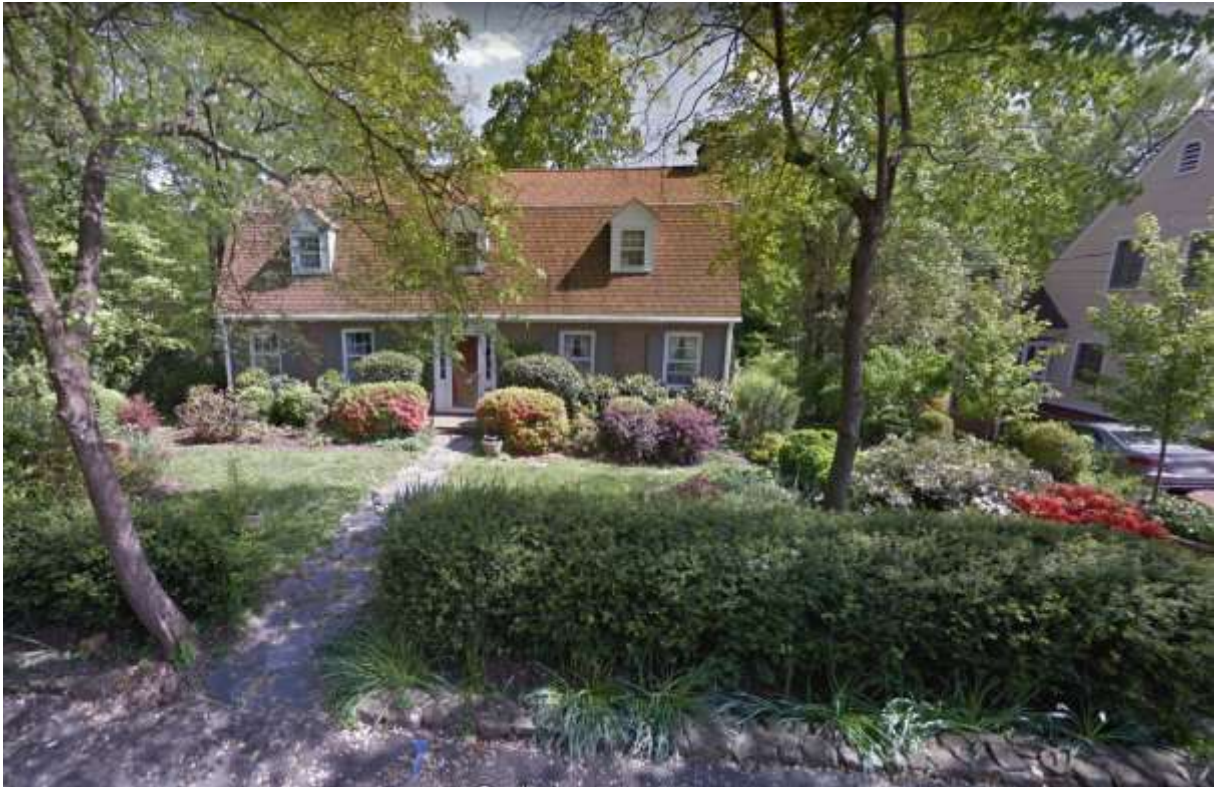
Figure 40 Existing vegetation blocking basement vents.
