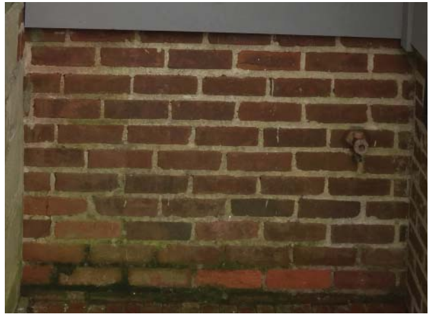
Existing running brick bond
