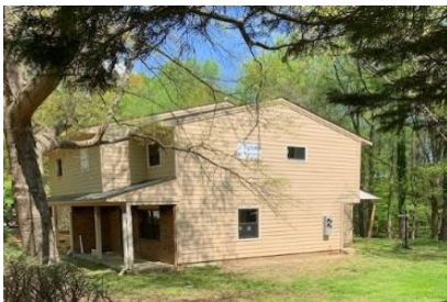
Oakwood, side of unit
