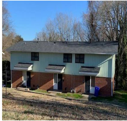
Reroofing of Craig/Gomains and Lindsay St. (19 buildings)
