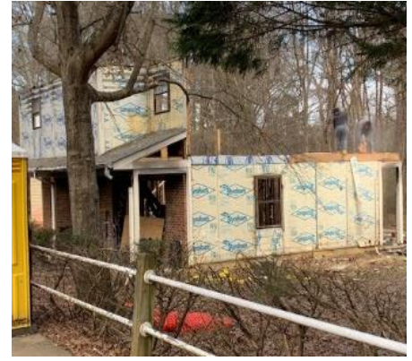
Rebuilding fire damaged Units (E-1 and E-2) Oakwood
