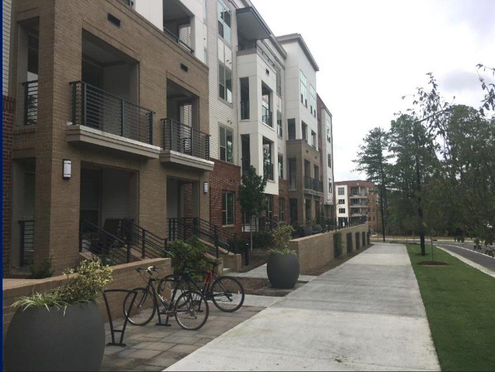
Completed Streetscape, Novus Ln Looking west from Legion Rd
