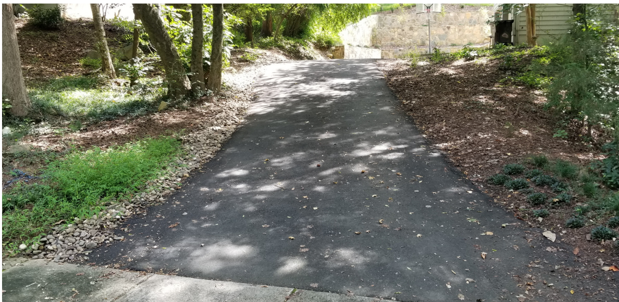
Photo 7 - Stone used for drainage scour protection in the neighborhood (left side of driveway)
