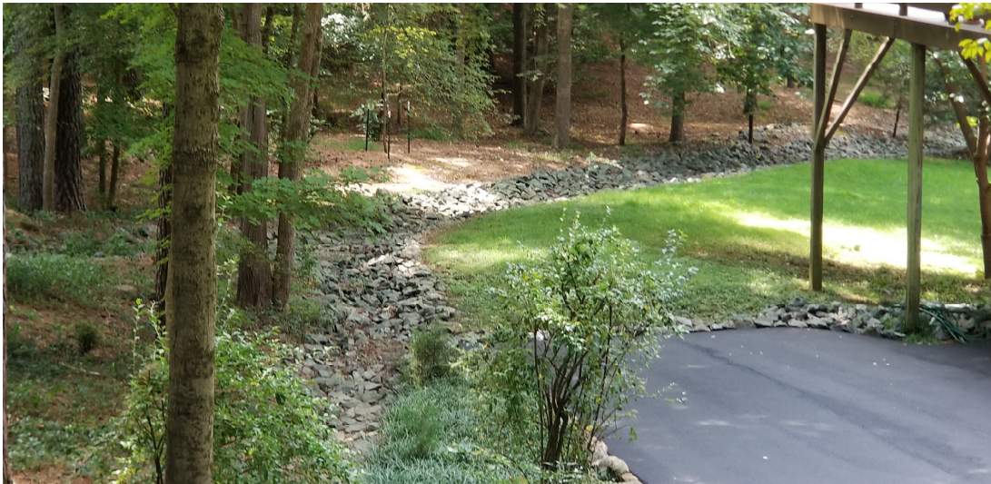
Photo 6 - Example of rock-lined drainage swale in the neighborhood
