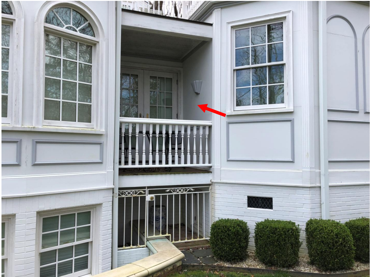
EXISTING PORCH TO BE FILLED IN WITH EXTERIOR WALL AND PANELING
