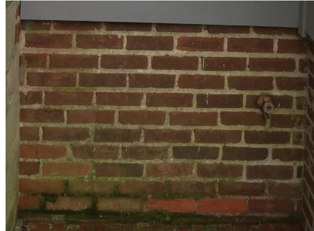
Existing running brick bond
