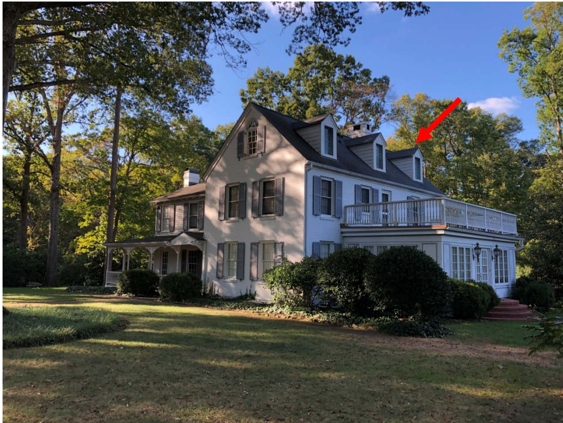
EXISTING DORMERS WITH ASPHALT SHINGLES
