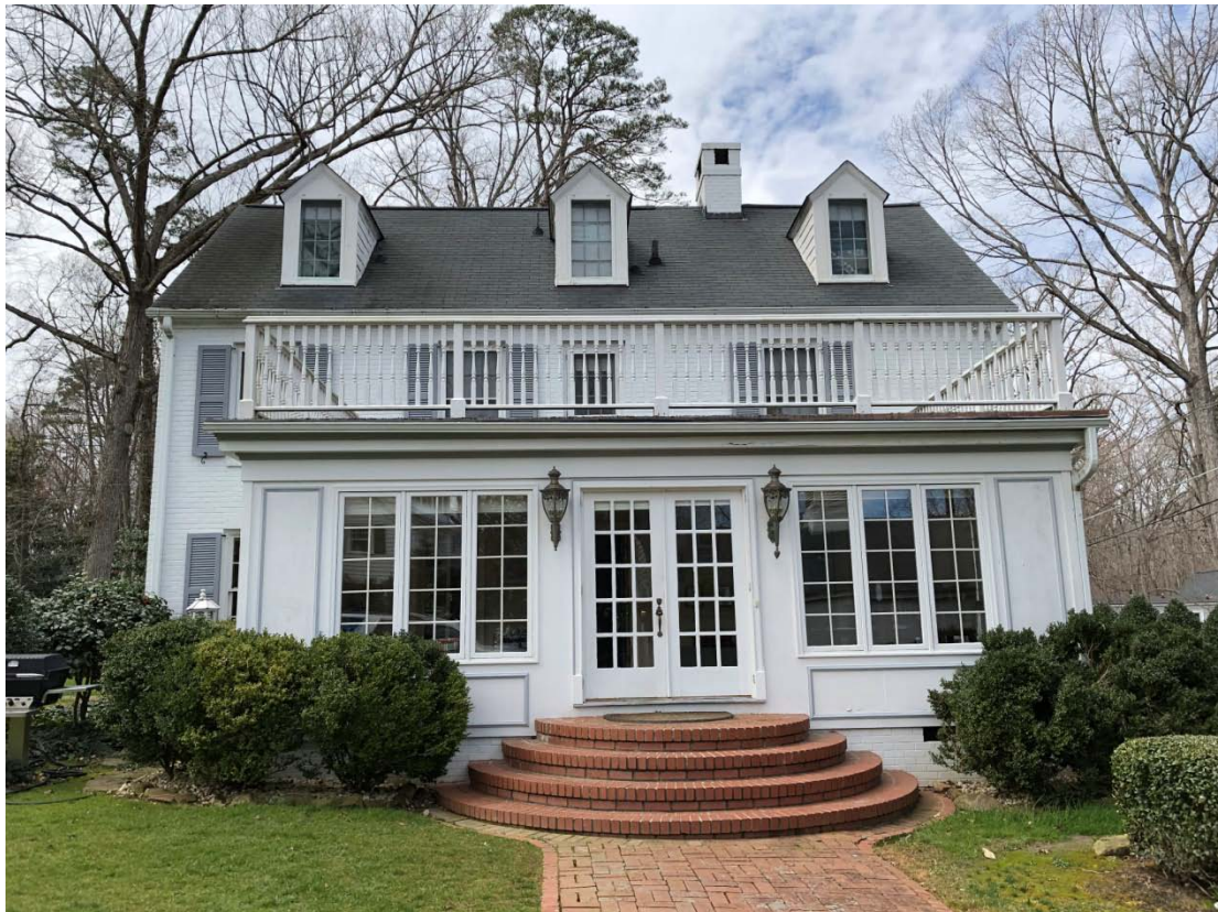
EXISTING DORMERS WITH ASPHALT SHINGLES
