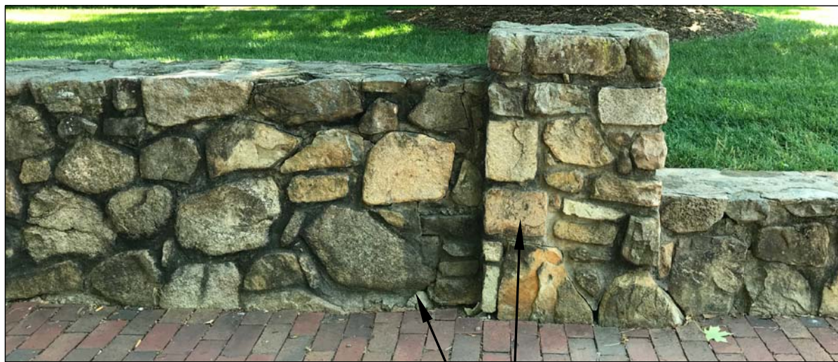
STONE WALL with low STONE PIERS Typical stone pier to extend approx. 4" above top of new stone wall. Native Chatham stone with <1" mortar joints
