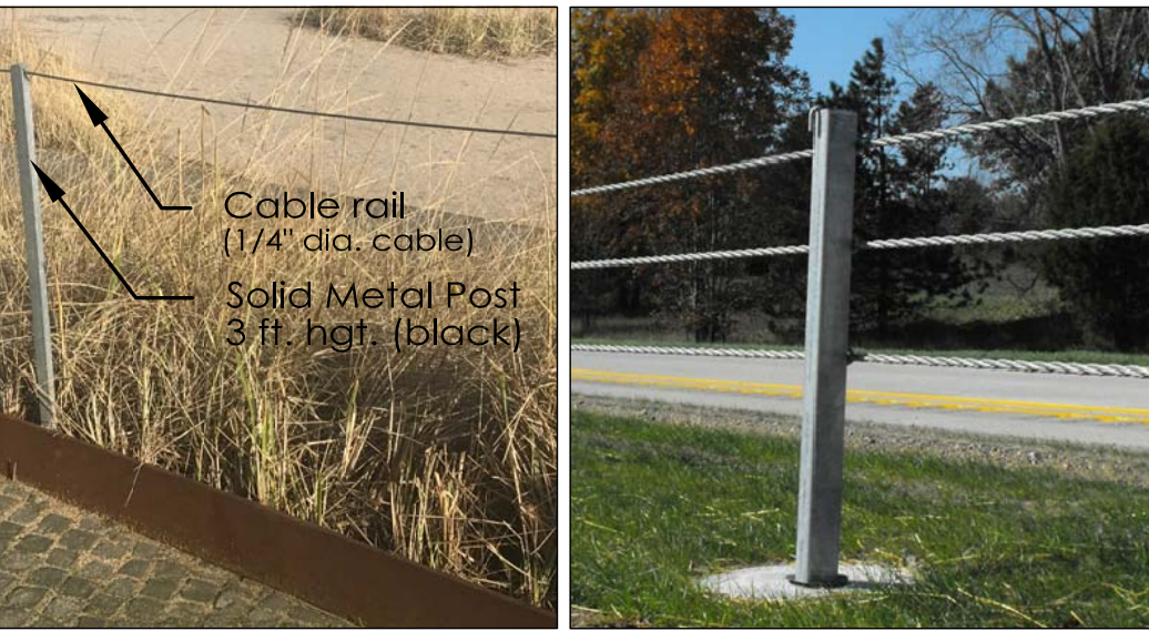
CABLE BARRIER RAIL and POST DETAIL precedent example of Cable Barrier Rail for pedestrian (left picture) and vehicular guard (right picture) rail situation.
