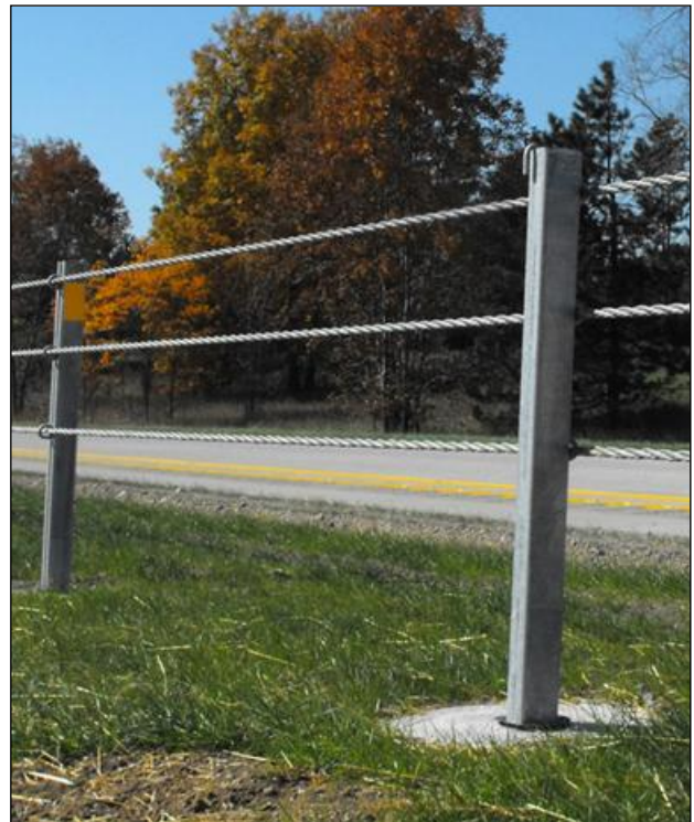
Examples of cable barrier rails and post details. The type on the left will be hidden within the existing holly hedge, and the type on the right will replace the existing guardrail near the dumpster.
