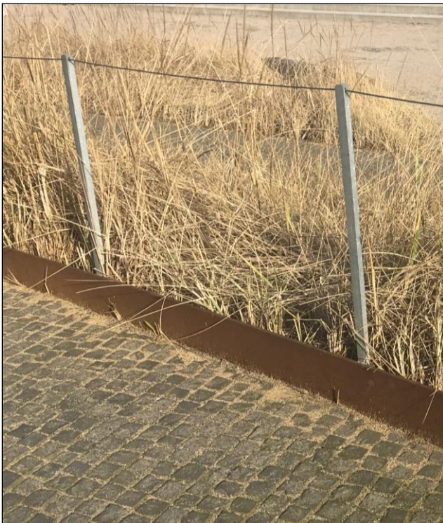
Examples of cable barrier rails and post details. The type on the left will be hidden within the existing holly hedge, and the type on the right will replace the existing guardrail near the dumpster.
