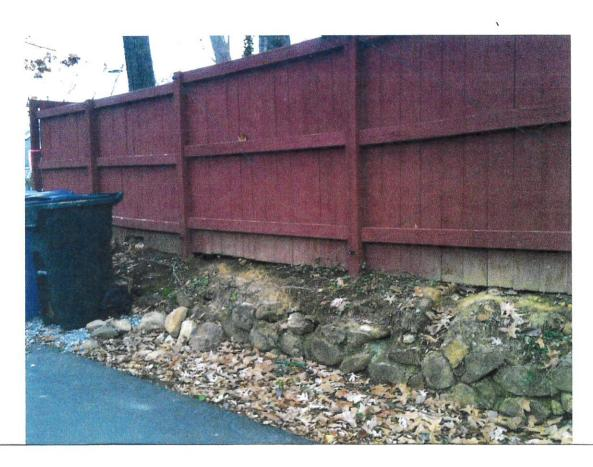
5. SECTION OF FENCE BEYOND ALCOVE THAT STILL REQUIRES REHABILITATION; DETERIORATING REMNANTS OF LOW STONE WALL VISIBLE AT BASE OF FENCE
