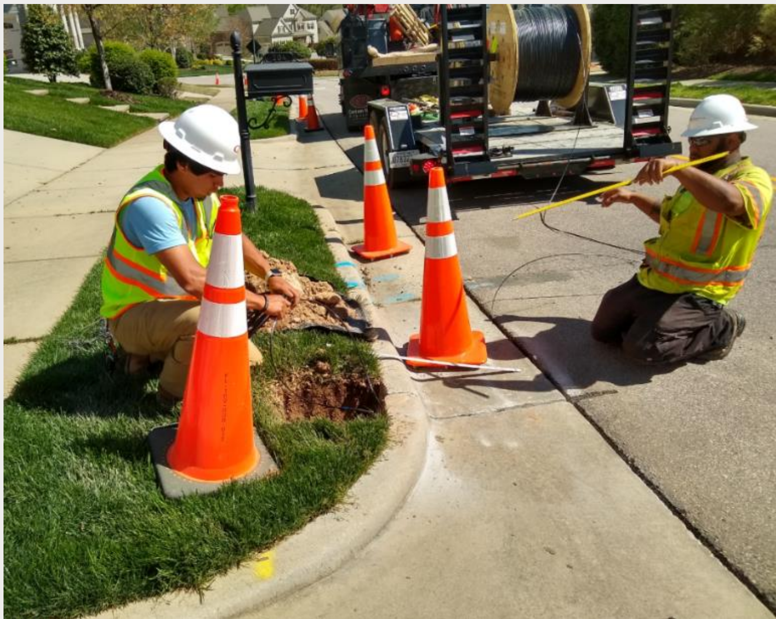
Shallow Depth – Laying in the Fiber
