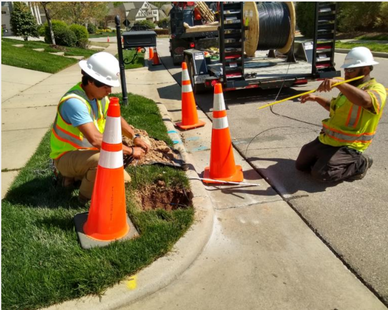
Shallow Depth – Laying in the Fiber
