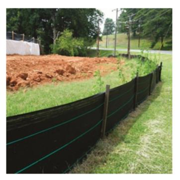
Photograph 1: Standard silt fencing
