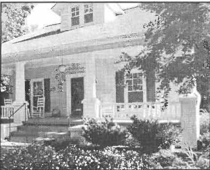
Six-over-one doublehung window sashes replaced inappropriate fixed single-pane glass panels during the sensitive rehabilitation of this bungalow.
