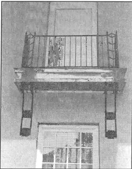
The shiny reflective surface of this newly installed copper balcony fascia will develop a greenish patina over time and does not require a protective coat of paint like the cast metal balustrade and brackets do.
