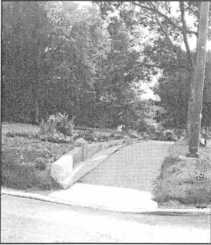
Where level changes or heavy traffic are a sidewalk safety or accessibility concern, brick pavers and concrete edging have replaced Chapel Hill gravel.
