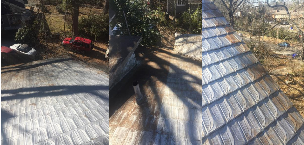
Aged metal panels with rust build up on front of property.
