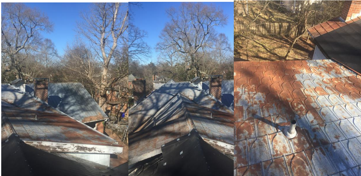
Roof view of roofing structures facing toward front and right of property of 305 McCauley st. Three total pipe boots on this side of the property that need to be replaced.
