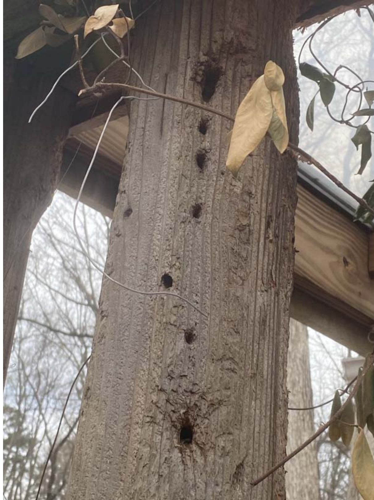
Pergola carpenter bee damage
