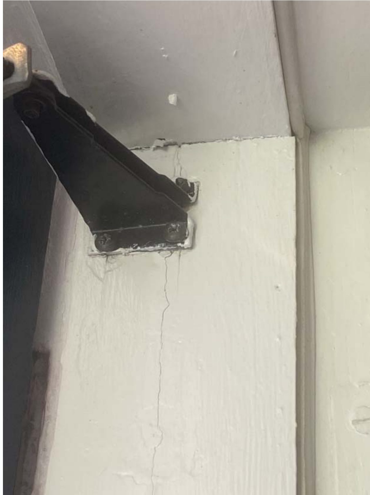
Storm door opener with split wood
