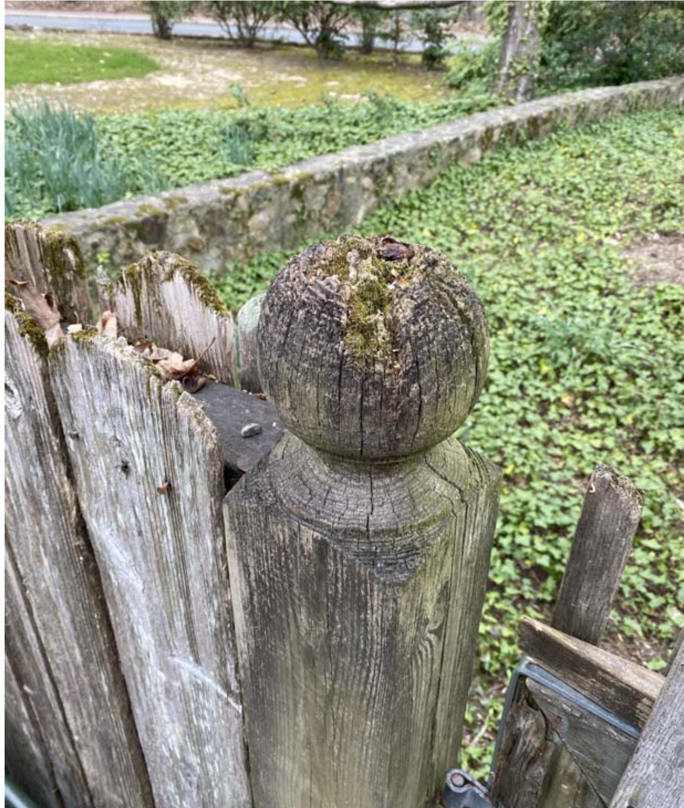
Existing fence and gate deterioration
