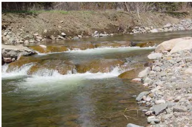
Figure 11-30 Cross vane/step-pool on the East Fork Piedra River, CO
