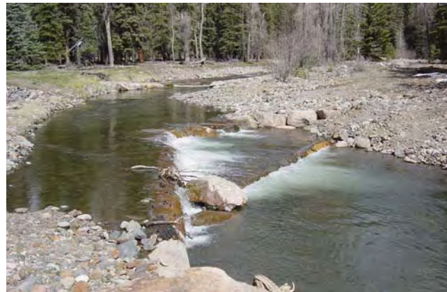
Figure 11-39 J-hook/log vane/log step with cut-off sill, East Fork Piedra River, CO
