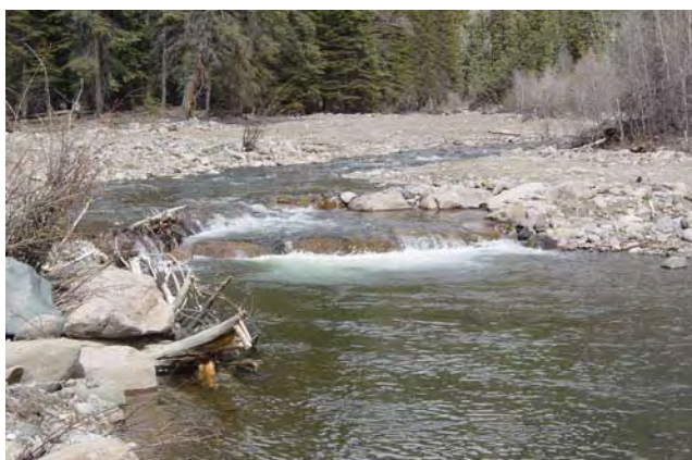
Figure 11-31 Cross vane/rootwad/log vane step-pool, converting a braided D4→C4 stream type on the East Fork Piedra River, CO
