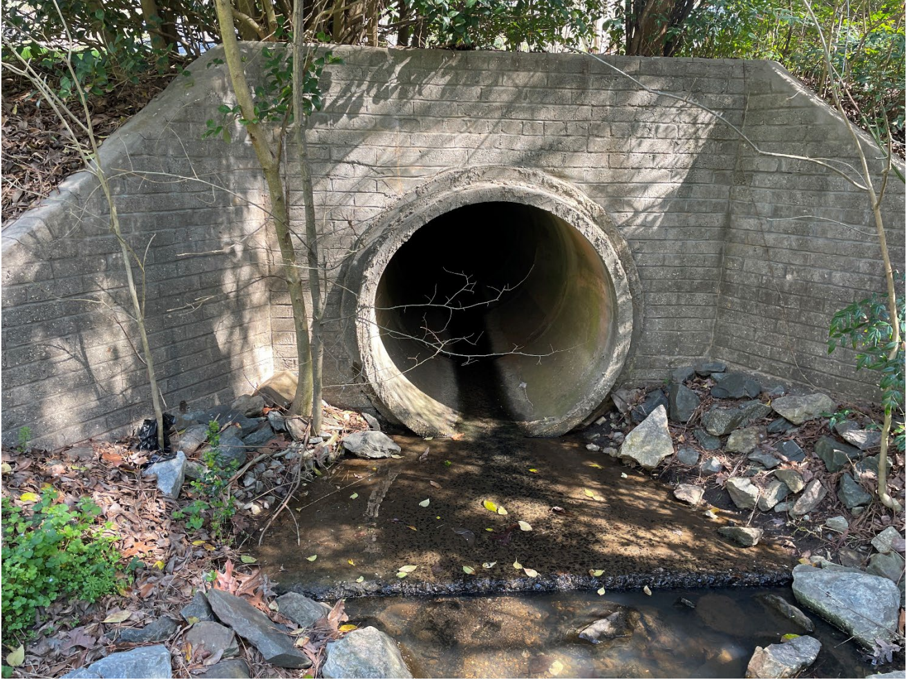
Photograph 8 – Pipe Culvert Outlet at Clover Drive
