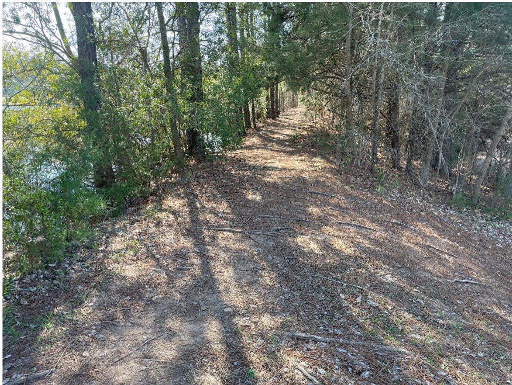
Photograph 2 – Dam Crest Facing East from West Abutment
