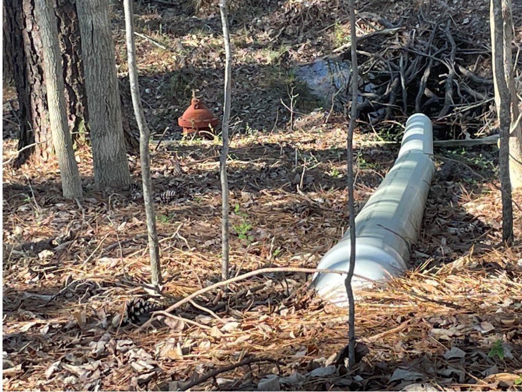
Photograph 5 – Overflow Outlet and Primary Outlet Valve from Dam Crest
