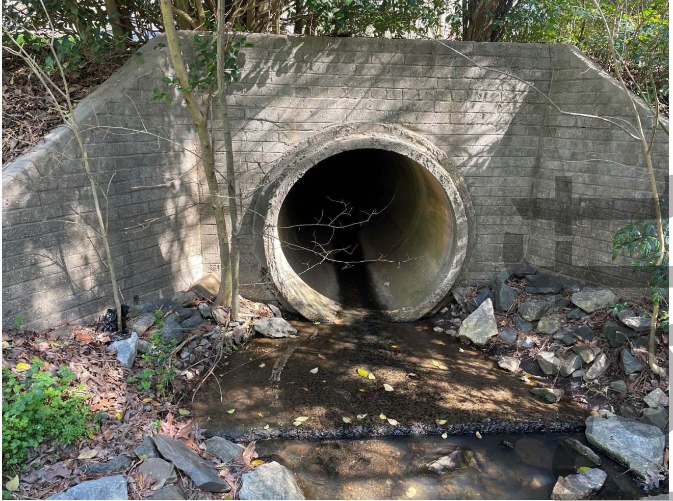
Photograph 8 – Pipe Culvert Outlet at Clover Drive
