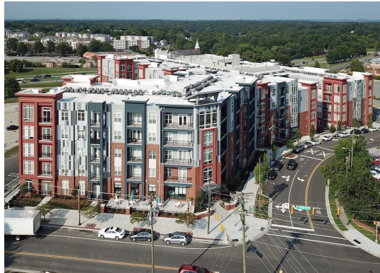
5-STORY | WRAP PARKING
