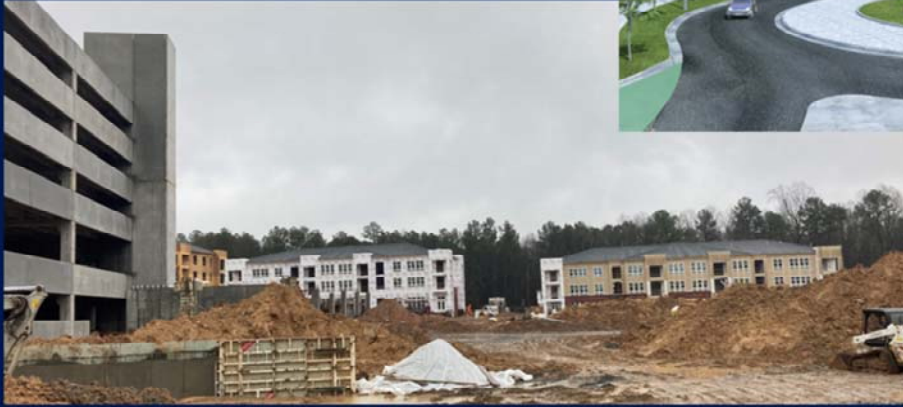
Construction Progress, view from northern site boundary
