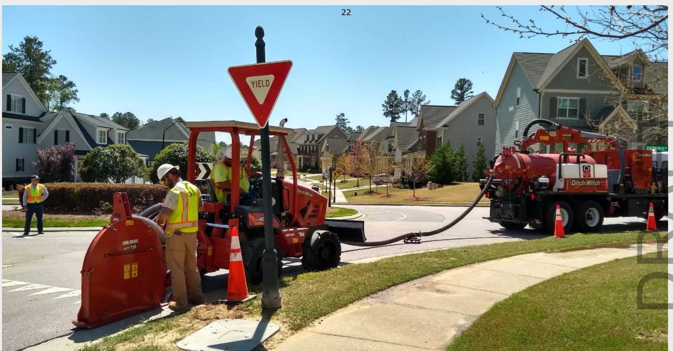
Worksite for New Installation Method - Shallow Depth Less Risk, Cleaner, Faster
