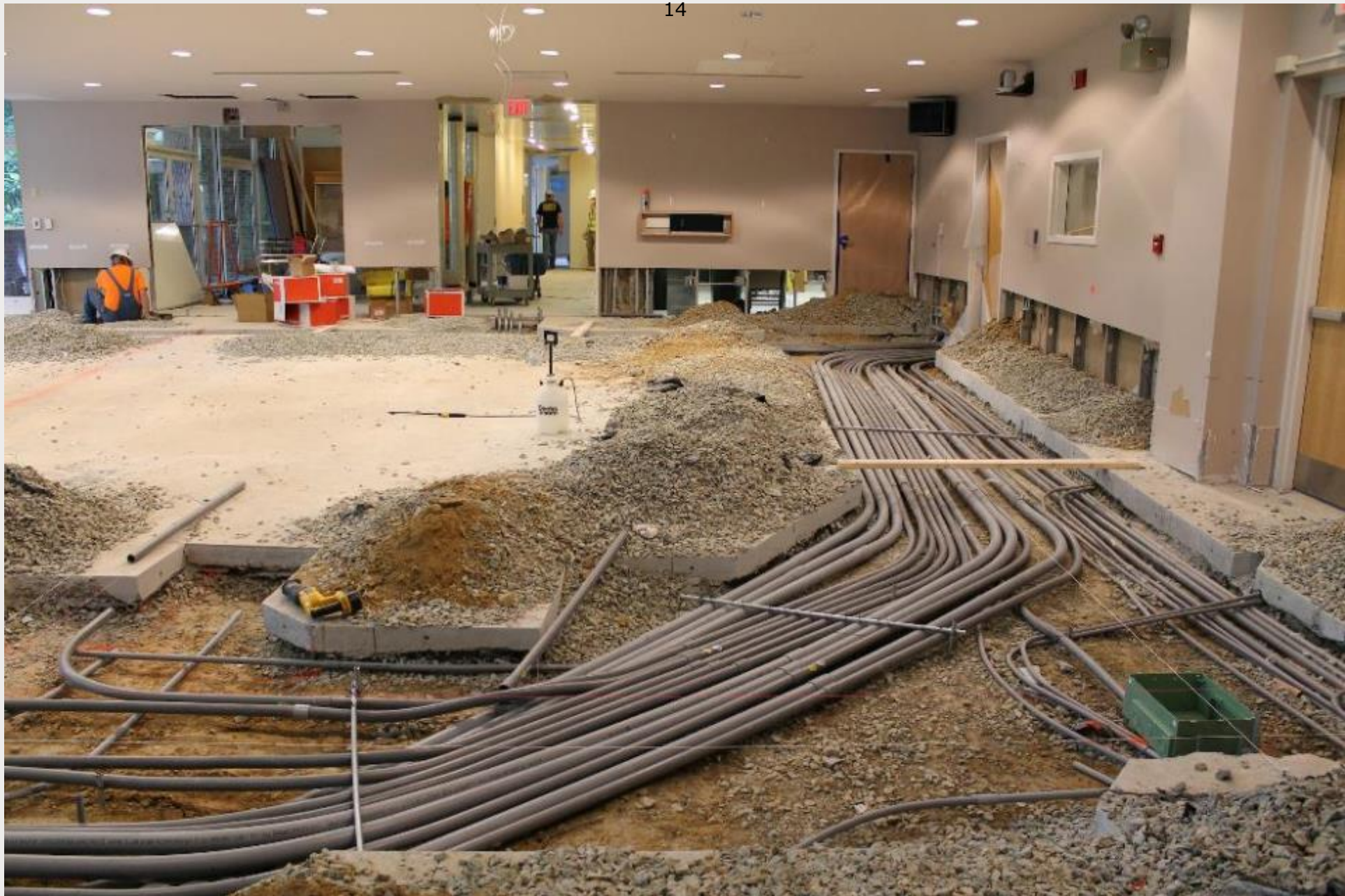
Council Chamber Construction (Several Years Ago)
