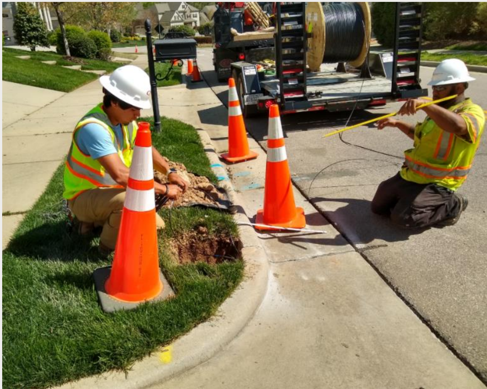
Shallow Depth – Laying in the Fiber
