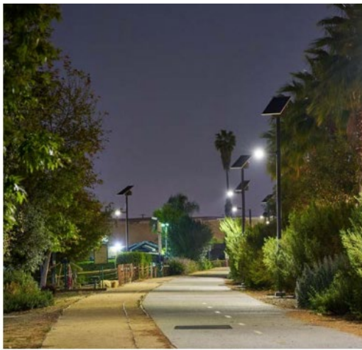
Solar Lighting on Whittier Greenway - Whittier, CA
