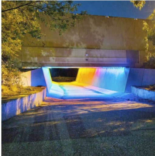
Colored Lighting at Larissa Underpass - Maroondah, Australia
