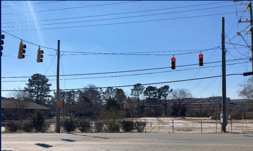
View of site preparation from northeast
