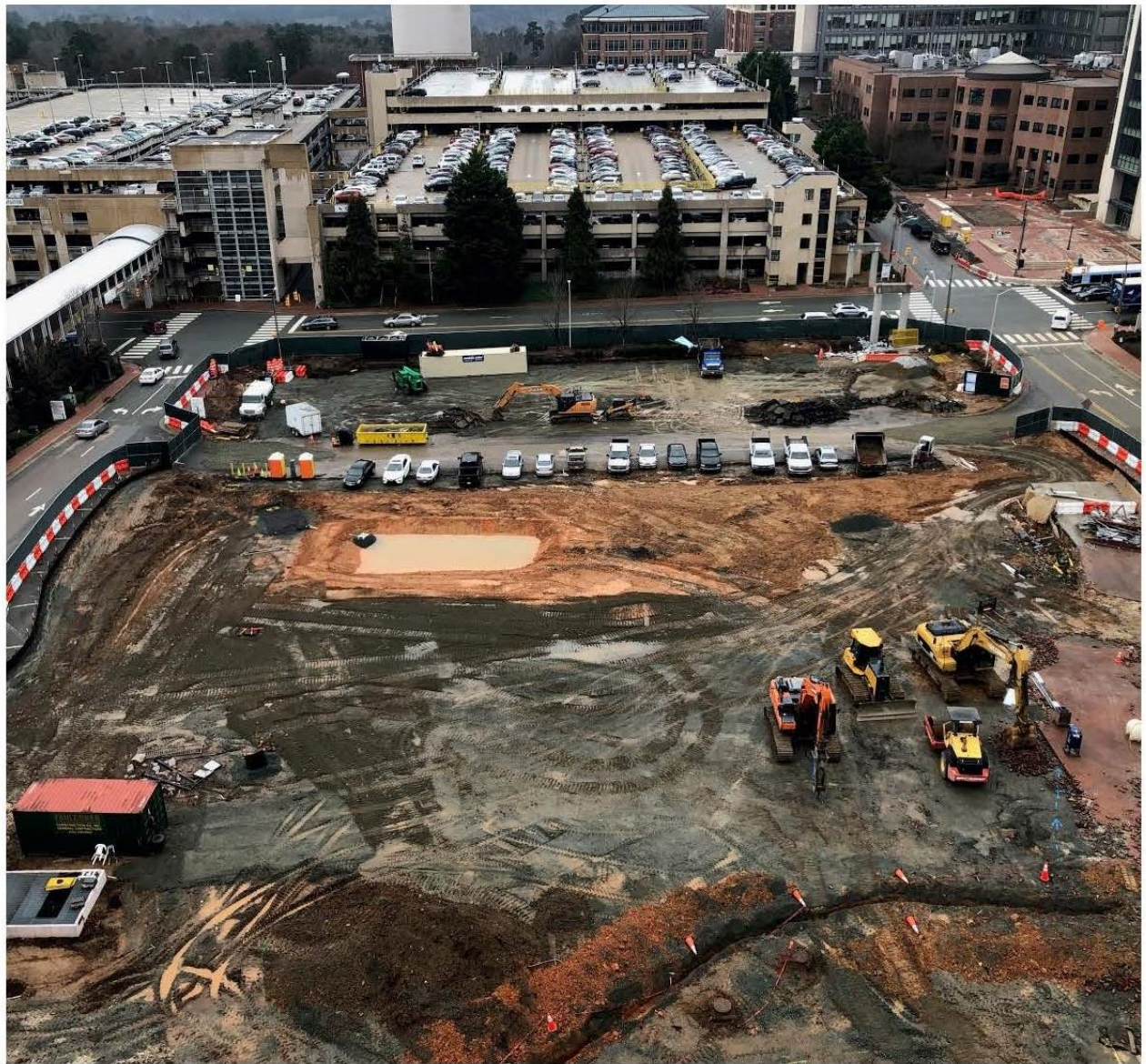
SITWORK PROGRESS VIEW TO THE SOUTH
