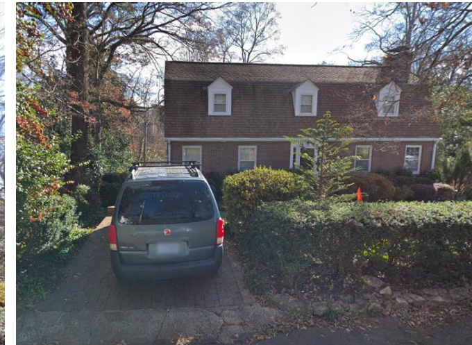
Image 2 | Existing Parking Pad
