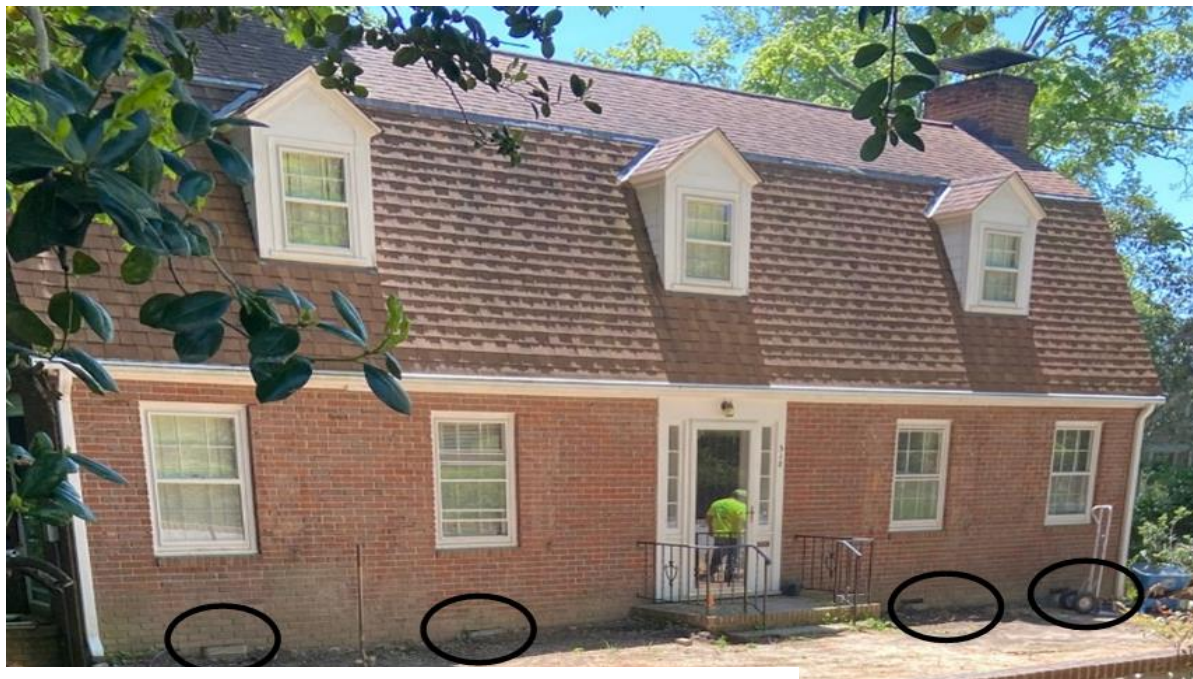
Image 2 | Cleared Front Yard – Basement Vents
