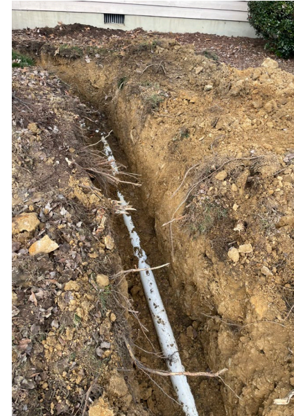
Install new PVC sewer lines
