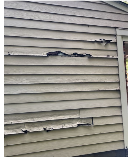
Install new siding
