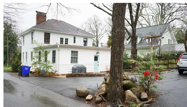
REAR OF EXISTING HOUSE AND BRICK PATIO / PARKING AREA
