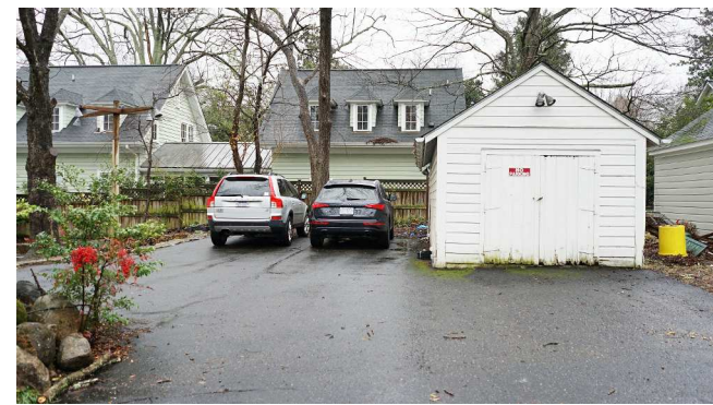
EXISTING STORAGE BUILDING TO BE DEMOLISHED
