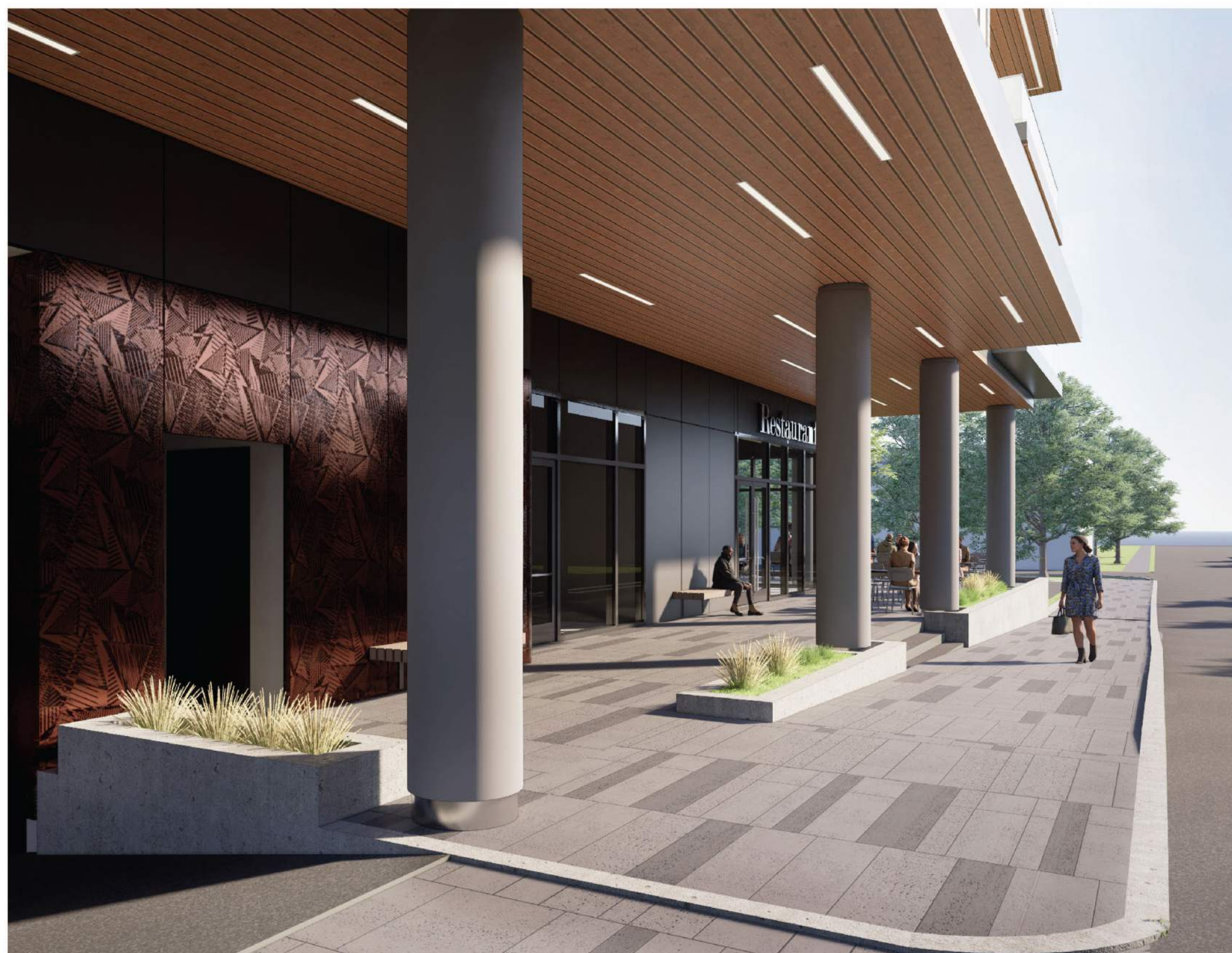
VIEW FROM NEW SIDEWALK ALONG ROSEMARY ST
