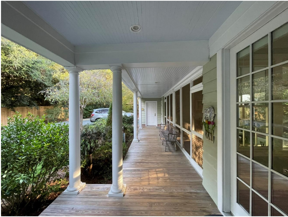
Open porch, looking south
