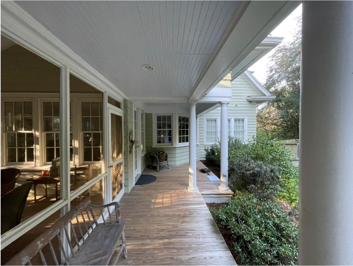
Open porch, looking north towards Rosemary Street
