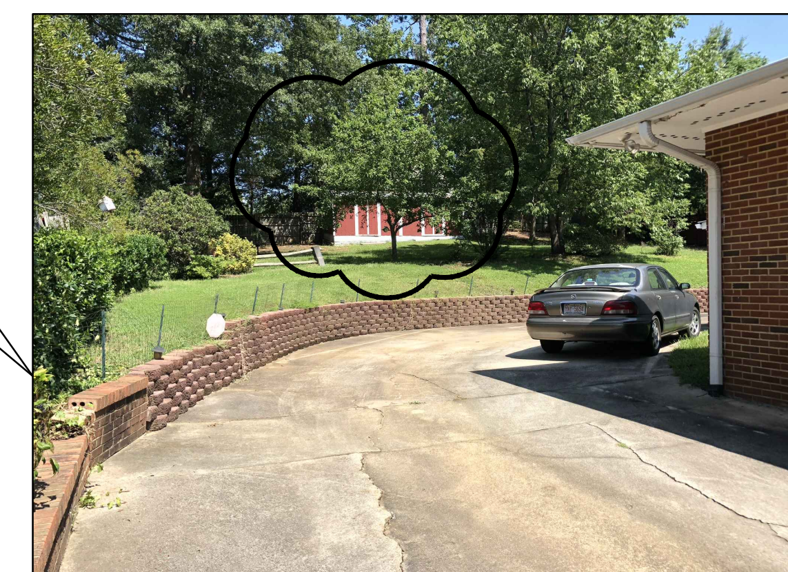
VIEW OF EXISTING SHED, RETAINING WALL & REAR LOT GRADE (ON CONCRETE DRIVE, LOOKING NORTH)
