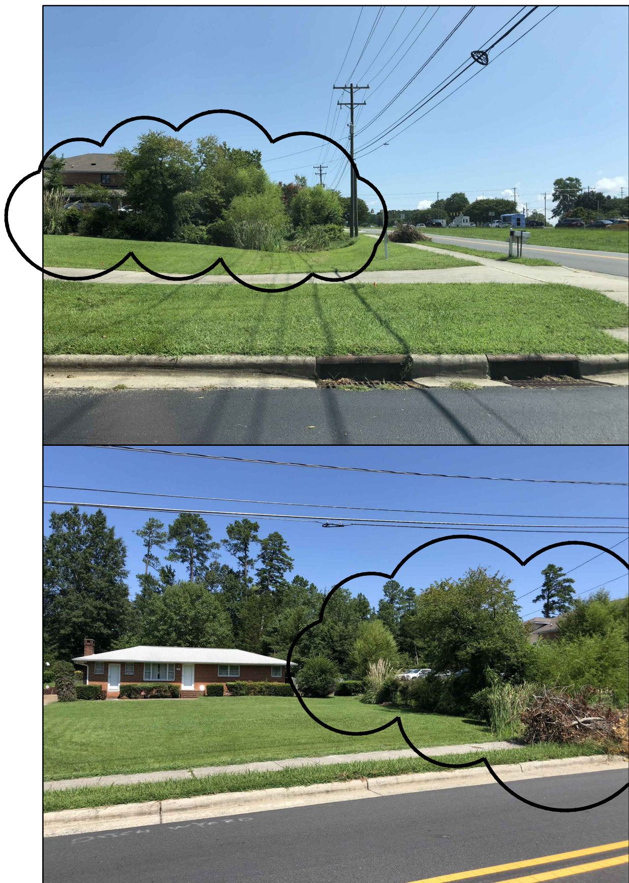
VIEW OF EXISTING DETENTION POND & BUFFER (ON DOBBINS, LOOKING EAST)
