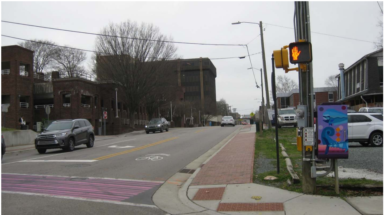
Street Scene along Rosemary Street Looking West
