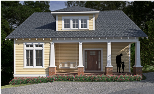
PROPOSED 412 W Patterson - 1.75 story Lot: .15 ac - Floor Area: 1,984 - Ratio: .33 Porch Eave - 11'-6" Dormer Eave - 18'-10"
