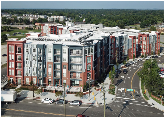
5-STORY | WRAP PARKING
