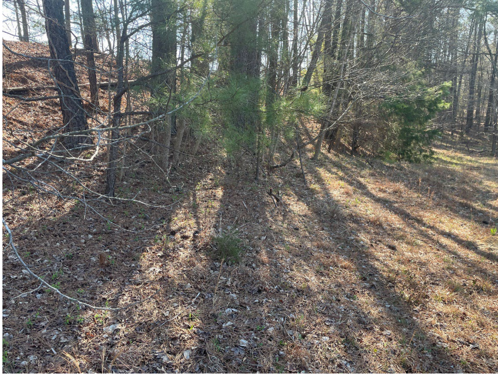
Photograph 3 – Downstream Face, Facing East from Western Groin
