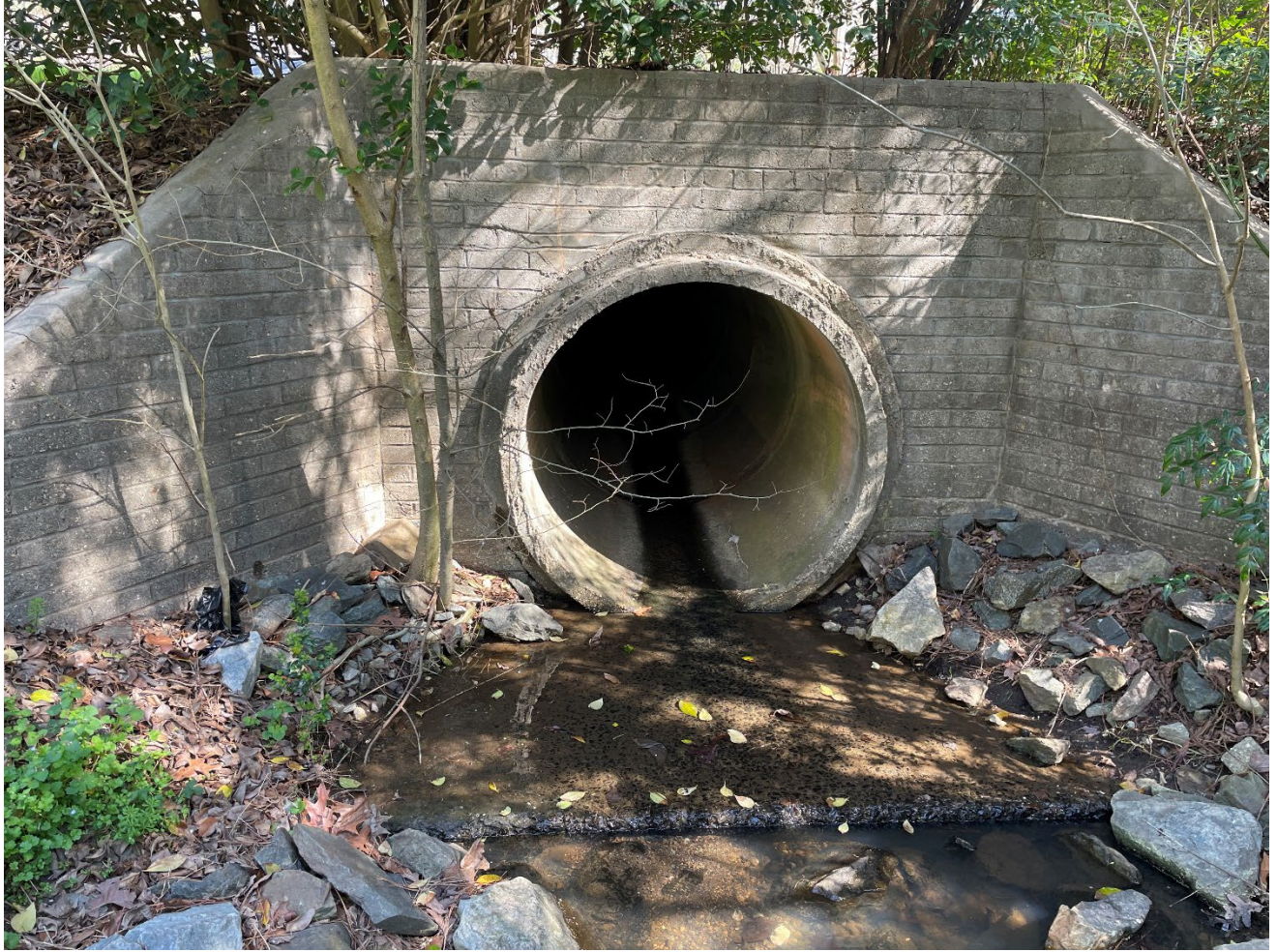
Photograph 8 – Pipe Culvert Outlet at Clover Drive
