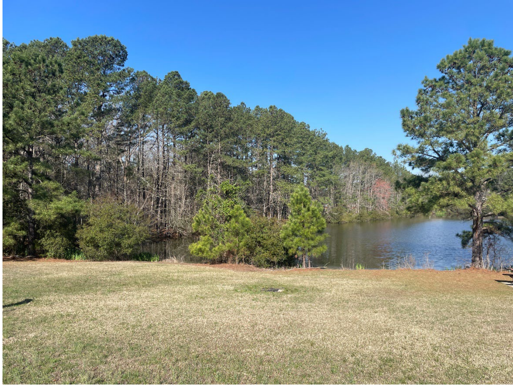
Photograph 1 – Impoundment Area and Upstream Dam Face from East Shore
