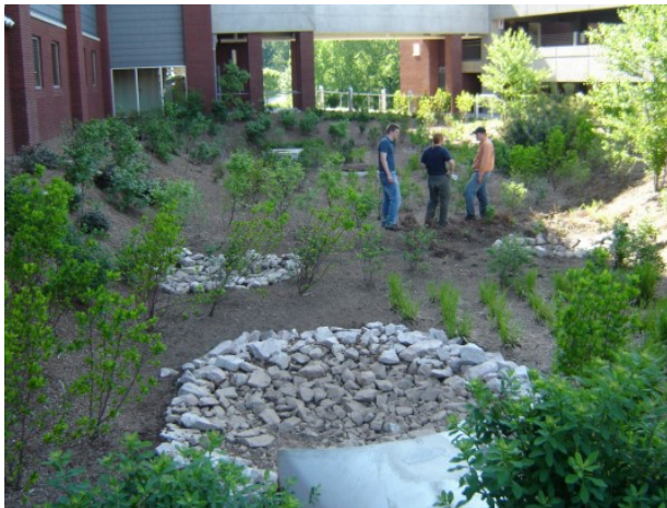
Bioretention facility NC DENR manual
