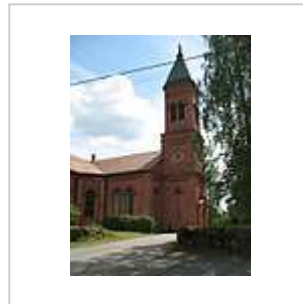
A 19th-century brick church in Loppi, Finland
