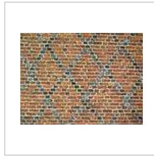
Decorative pattern made of strongly fired bricks in Radzyń Castle (14th century)
