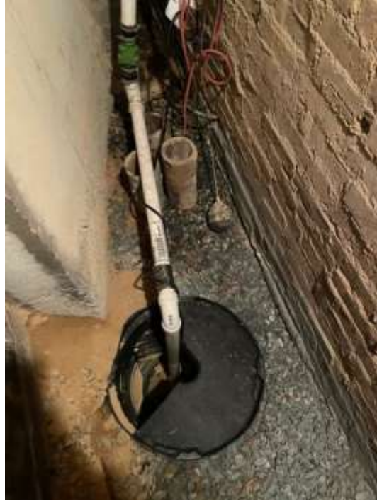
Figure 6 -Sump pump installed to remove water and gravel area which never dries out.
