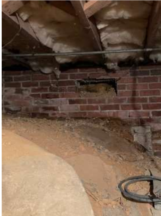
Figure 2 - Brick on soil in the northwest corner
