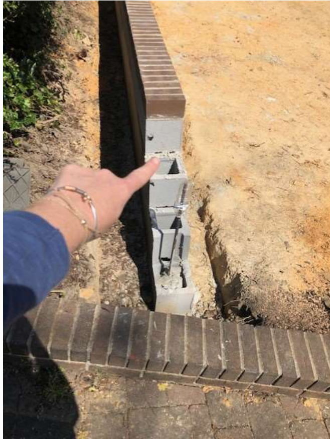
Figure 8 - Concrete Brick Wall – Rebar every 2'
