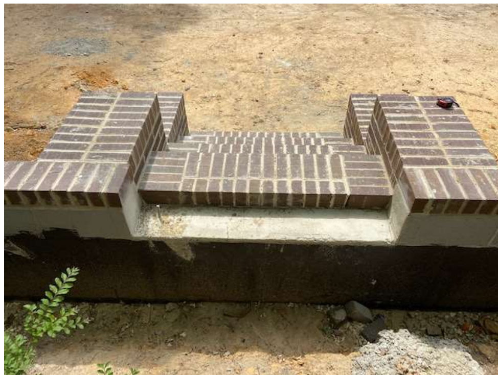
Figure 9 - Applied Masonry Sealer on the back of new concrete brick wall
