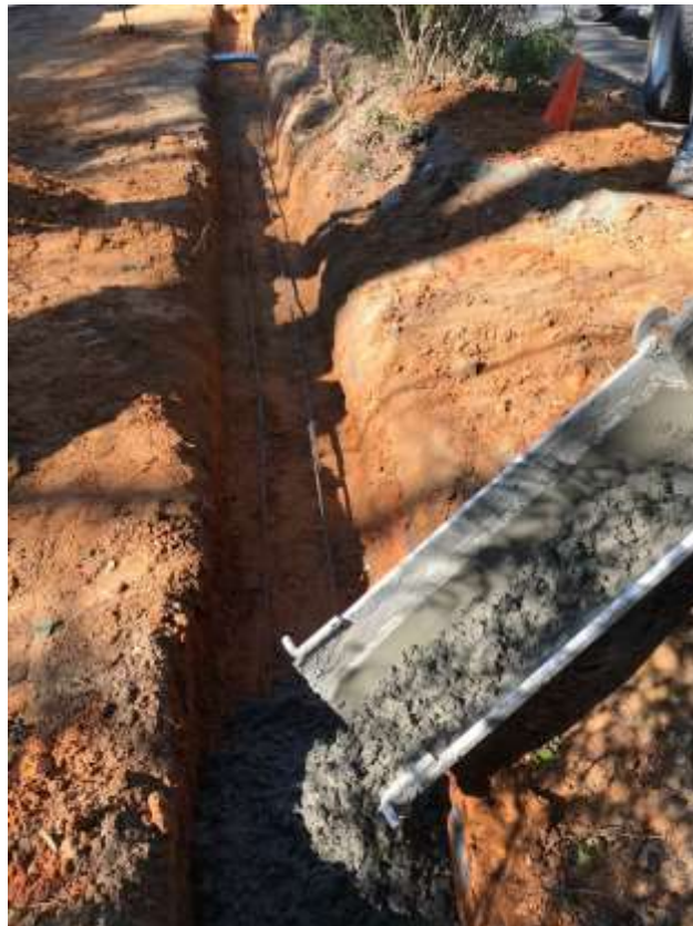
Figure 7 - Block wall footer being poured.
