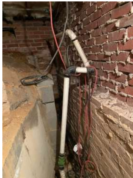
Figure 3 - Block amendment to hold back soil.
