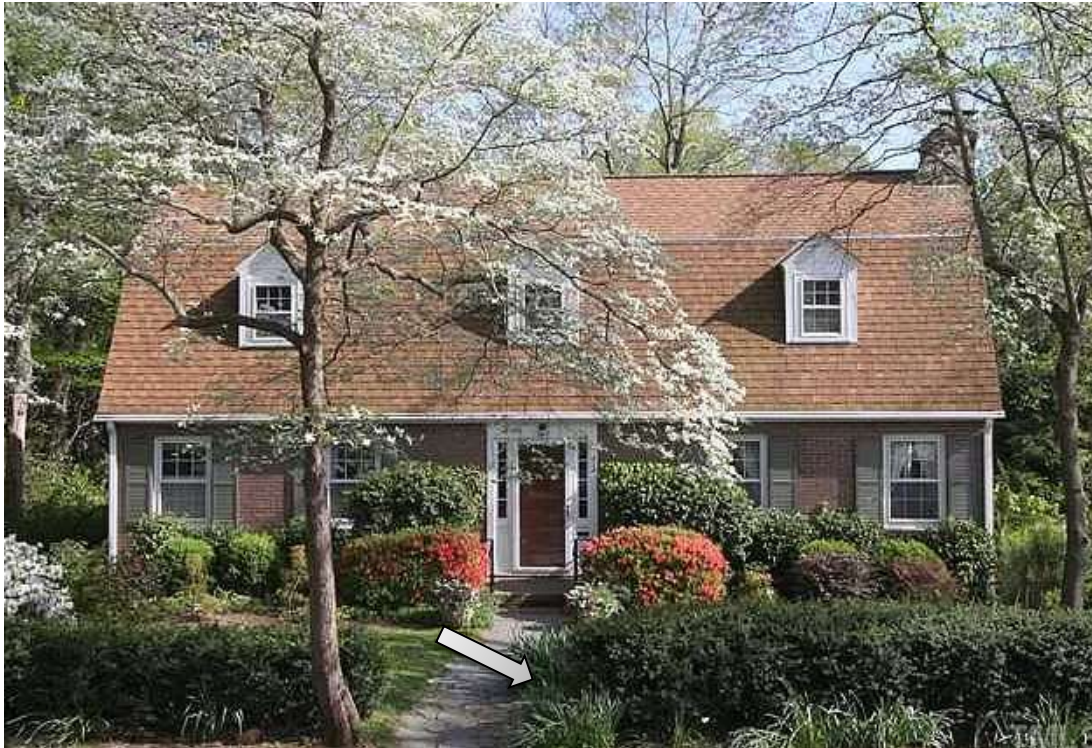
Figure 38 - View of existing slate to be replaced.
