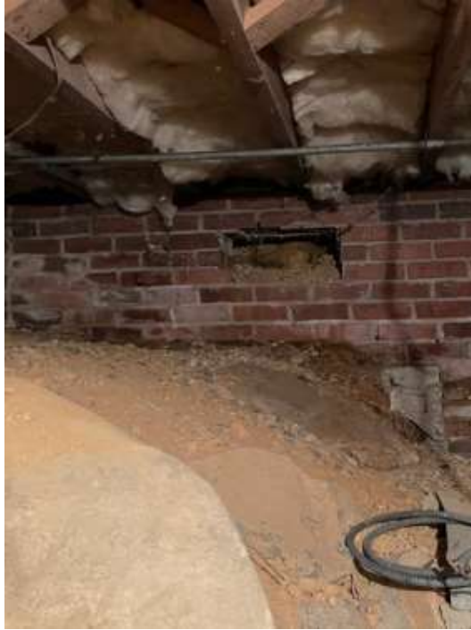
Figure 4 Soil thru vents next to soil that has started to cave in.
