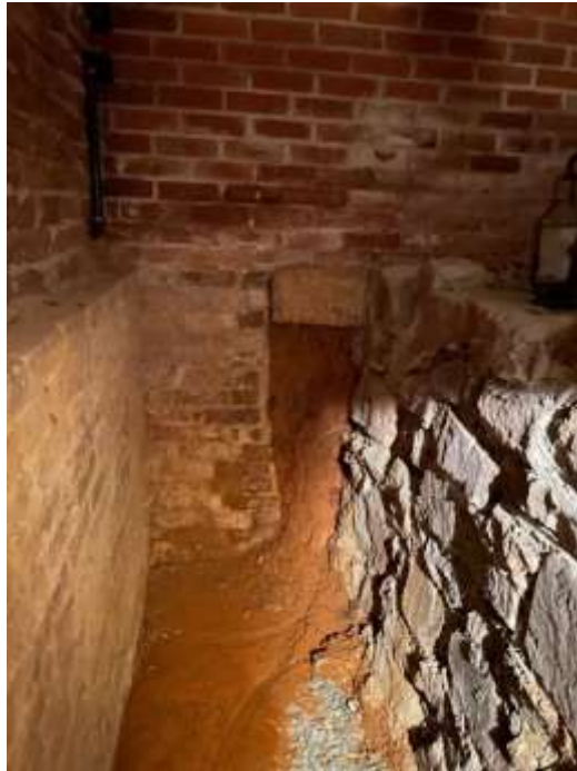
Figure 5 - Area where soil is collapsing - Water runs into the space during every storm and is heavy during heavier times. It is now just starting washing in.
