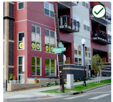
Figure 3-50 Design a building to step with the existing topography of a site.
