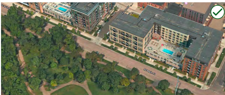
Figure 4-4 Locate the taller portion of a structure away from neighboring residential buildings of lower scale or other sensitive edges.
