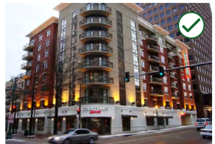
Figure 4-44 Install exterior lighting that will enhance the public realm and improve the pedestrian experience.
