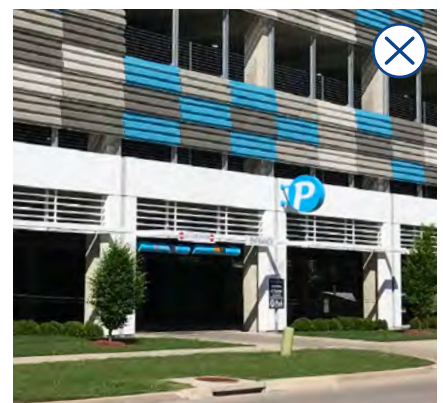
Figure 3-35 Provide an active use at the sidewalk edge when parking in a structure occurs at the street level on a primary street.
