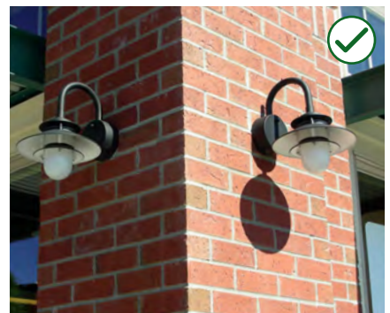
Figure 4-47 Use shielded and focused light sources to prevent glare and light pollution.
