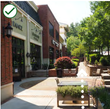
Figure 3-52c Consider locating a sloped sidewalk adjacent to stepped hardscape areas in order to maintain ADA access.
