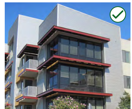
Figure 4-38 Architectural metal may be considered as a primary building material for design alternatives on building walls.
