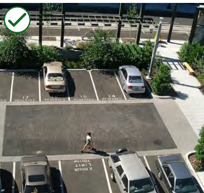
Figure 3-63 Incorporate Low Impact Development (LID) principles, such as stormwater planters and permeable pavement, to mitigate stormwater impacts.
