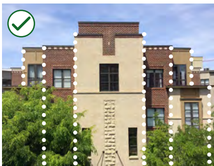
Figure 4-7 Provide vertical articulation in a larger building mass to establish a sense of scale.
