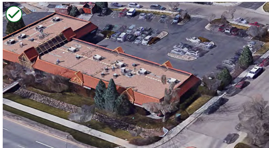
Figure 3-32 Locate a surface parking lot so it will minimize gaps in the continuous building wall of a commercial block.
