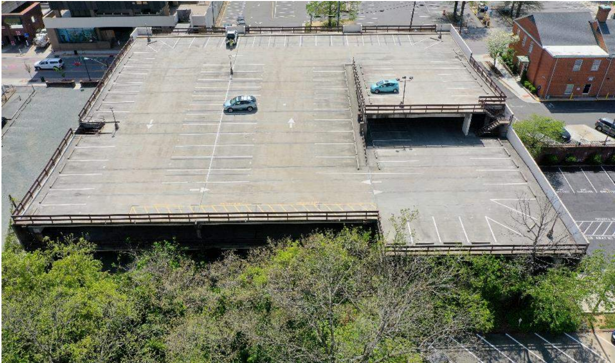
Photo 4 –Northern elevation of existing parking deck
