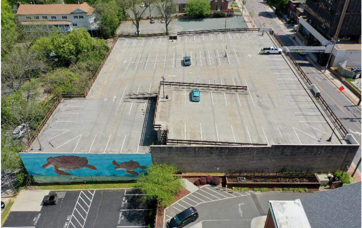
Photo 2 –Western elevation of existing parking deck
