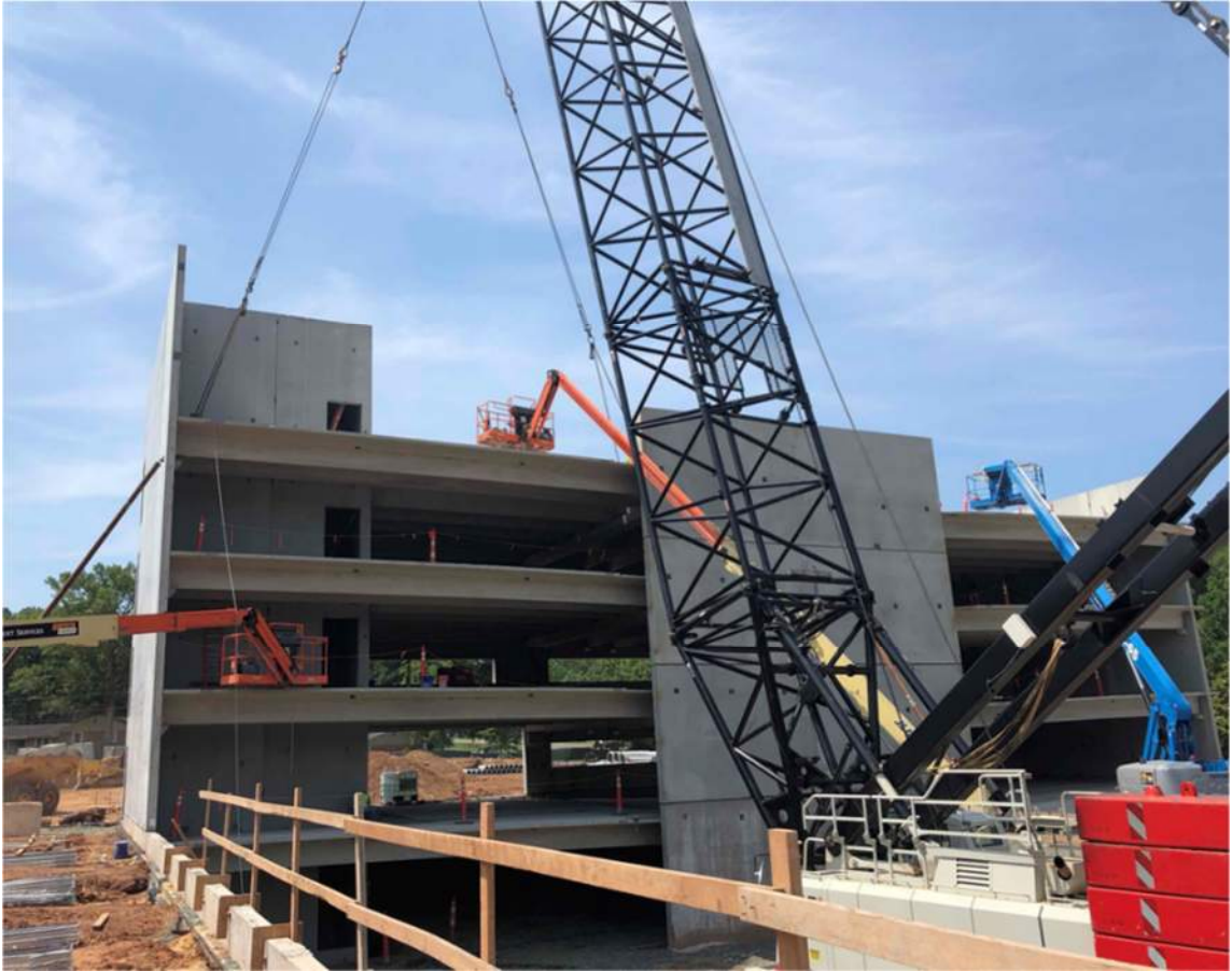
Figure 6 – Example of Crane within parking deck footprint placing a double-tee.
