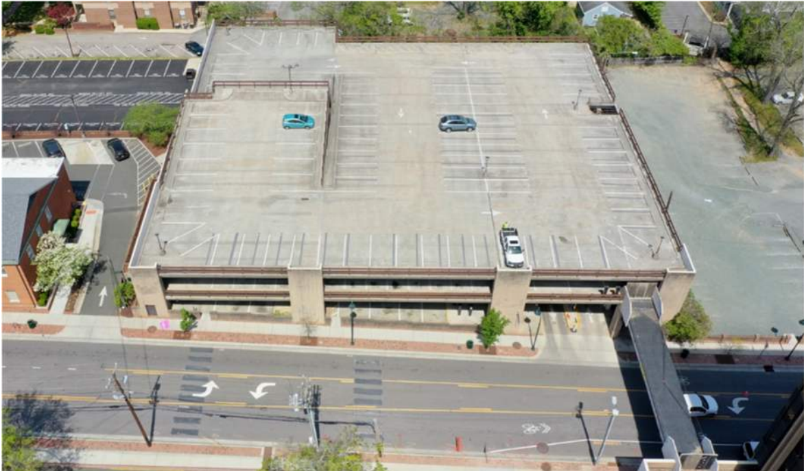
Photo 1 – Existing 3-Story Parking Deck
