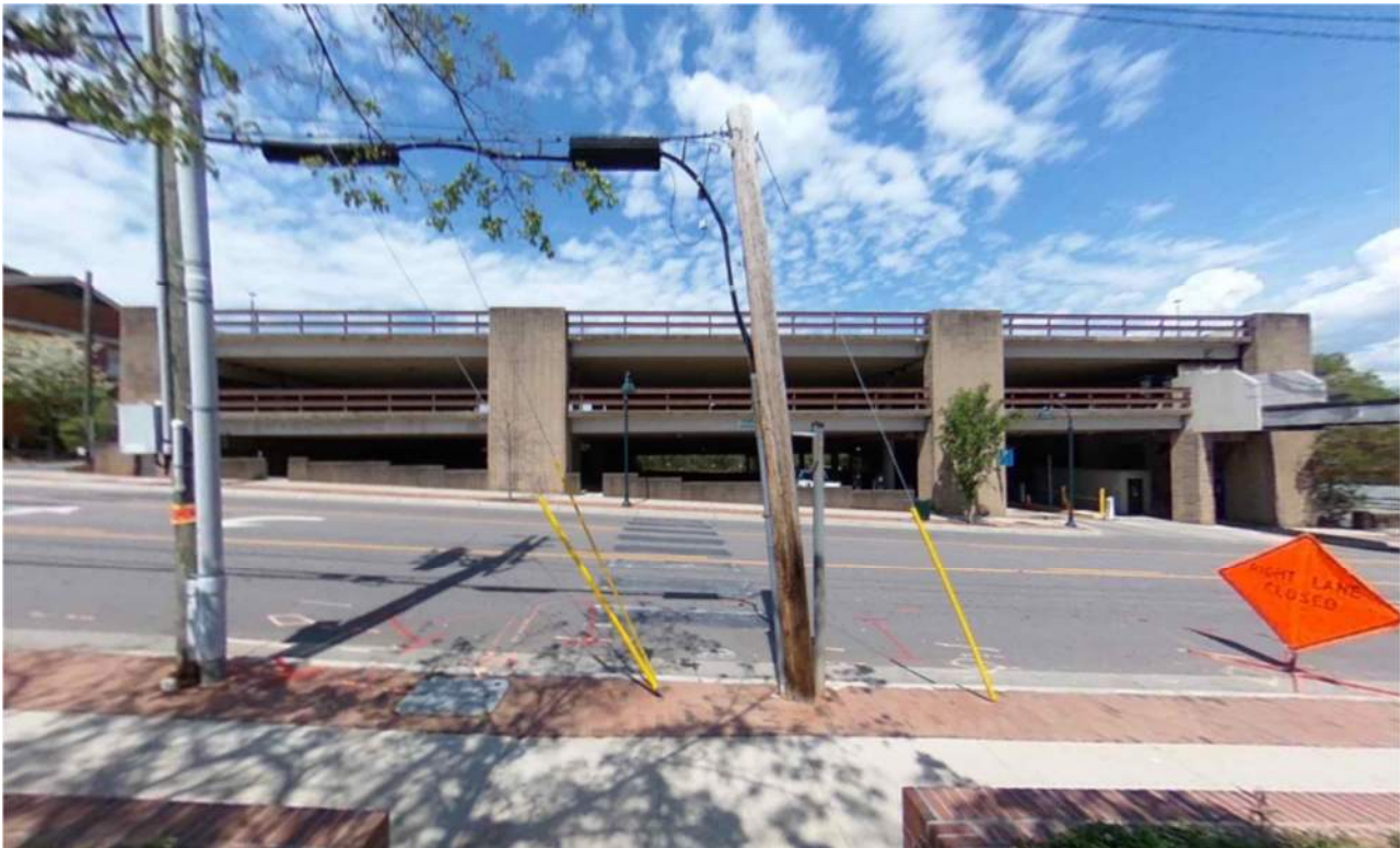
Photo 6 – View of Rosemary Street and south elevation of existing deck.
