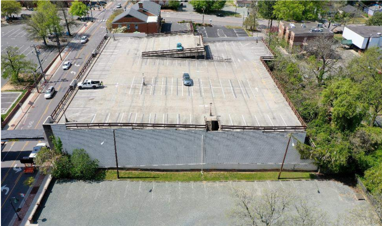
Photo 3 – Eastern elevation of existing parking deck
