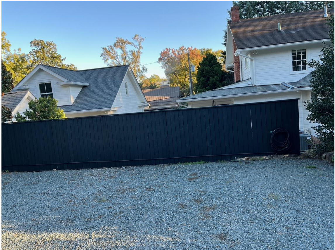
This is the privacy fence, and the picture above is of the fence and entrance to my house and pool.
