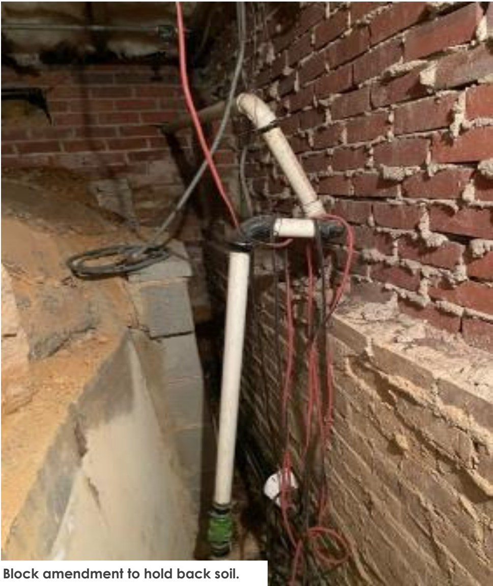
Area where soil is collapsing - Water runs into the space during every storm and is heavy during heavier times. It is now just starting washing in.
